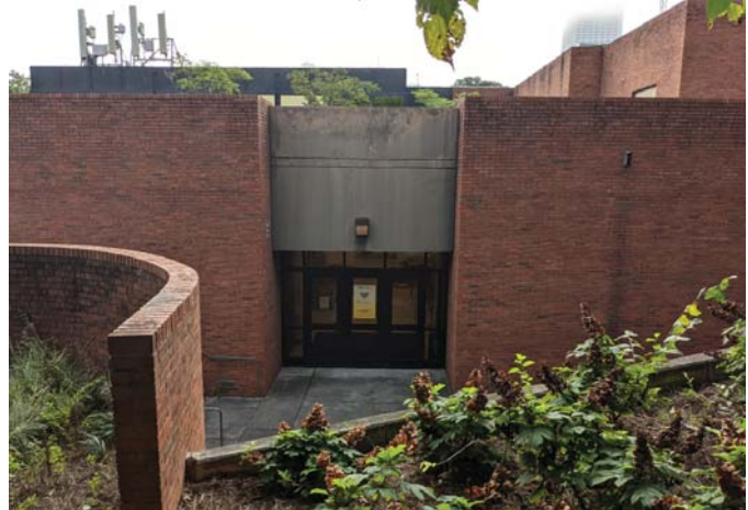
Figure 18: “New” Rich’s below-grade west entrance.
