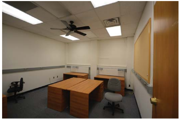
Figure 27: Interior office in the Calculator Building showing typical finishes and conditions. Note the boarded up exterior windows.
