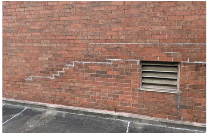
Figure 29: 1971 Rich building wall with sealant in mortar joints.
