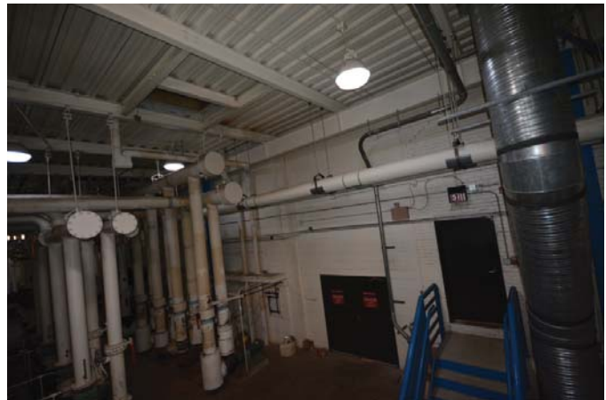
Figure 24: Interior of the Rich Chiller Plant showing exposed, painted structure.
