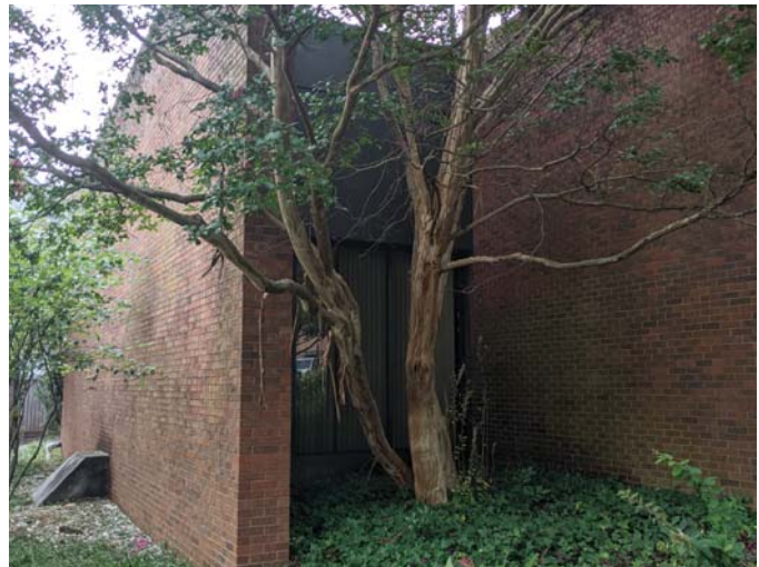
Figure 21: Fixed window at the ground floor of New Rich.
