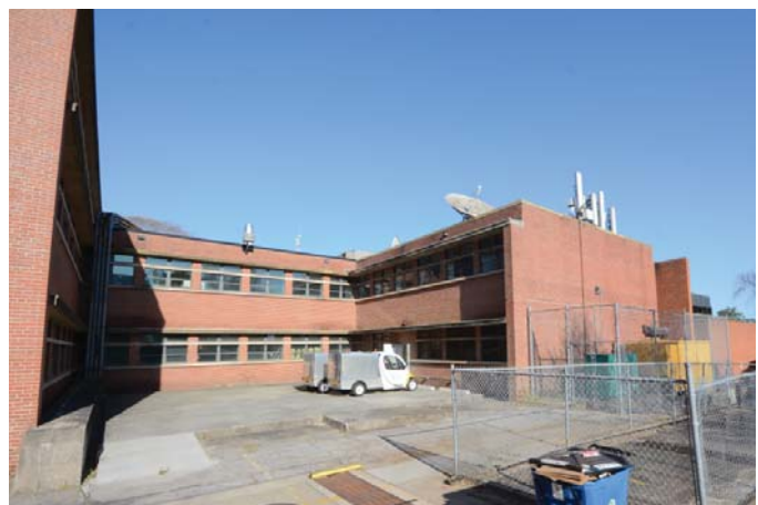
Figure 11: View of Hinman Research building addition wing (center) and Calculator Building (right), looking northwest.
