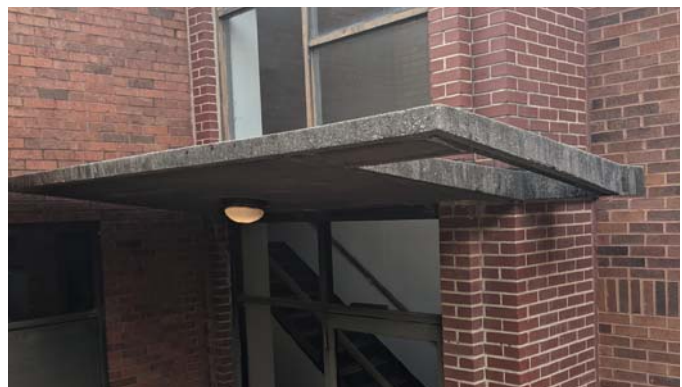
Figure 26: Concrete canopy at west entrance to Old Rich.
