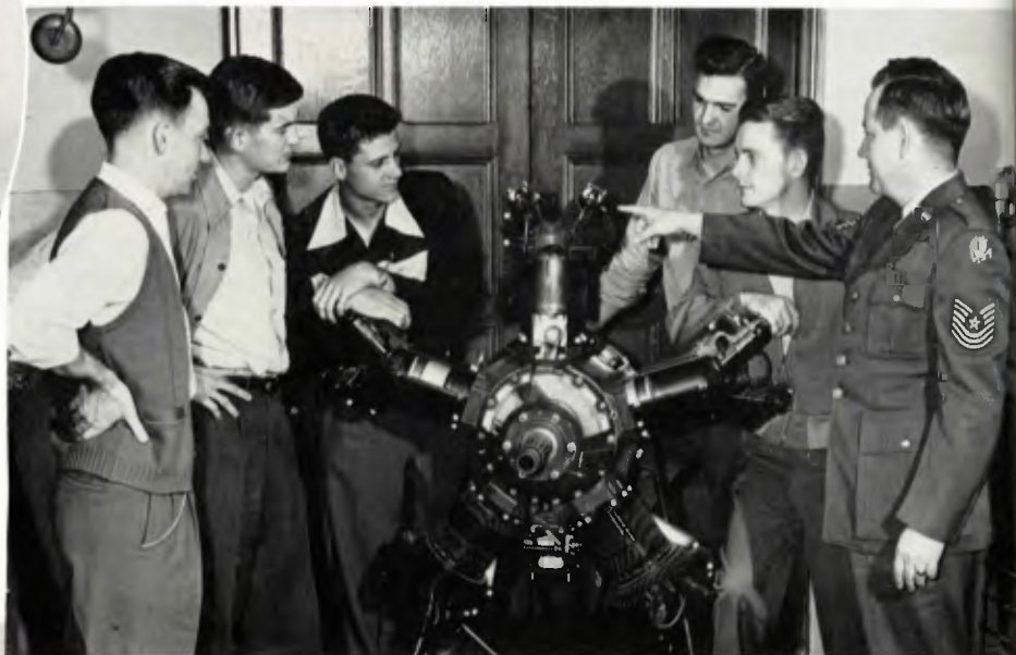
Engine inspection procedure.
