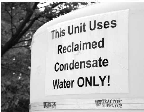
Tanks located around Tech buildings help to capture thousands of gallons of water generated by campus air conditioning units.
