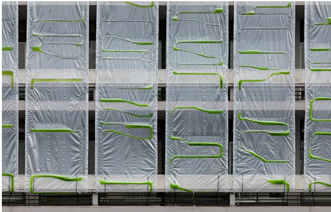
Figure 8 - Main façade of Printworks building at Dublin Castle presented in Climate Innovation Summit 2018
