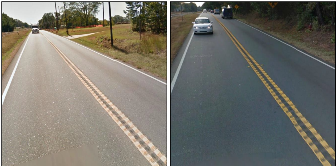
Figure 11. Project 0006693, SR 14 Details (clockwise from top left): Map [22-24], Location within Georgia, MP 21 Facing South [4, 21], MP 27 Facing North [4, 21]
