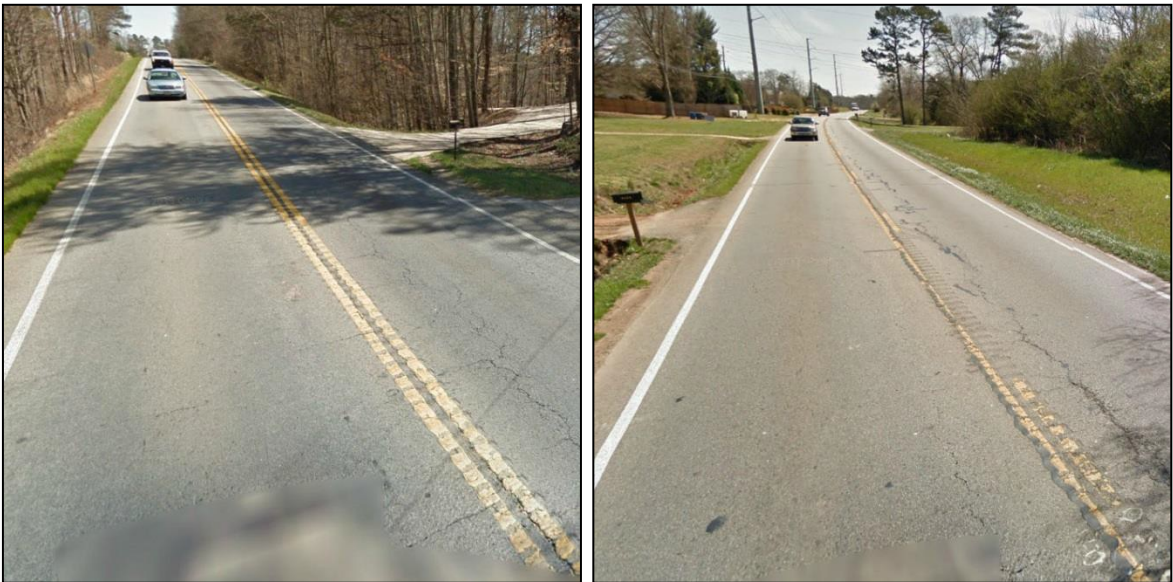
Figure 13. Project 0006945, SR 369 Details (clockwise from top left): Map [22-24], Location within Georgia, MP 10 Facing East [4, 21], MP 1 Facing East [4, 21]
