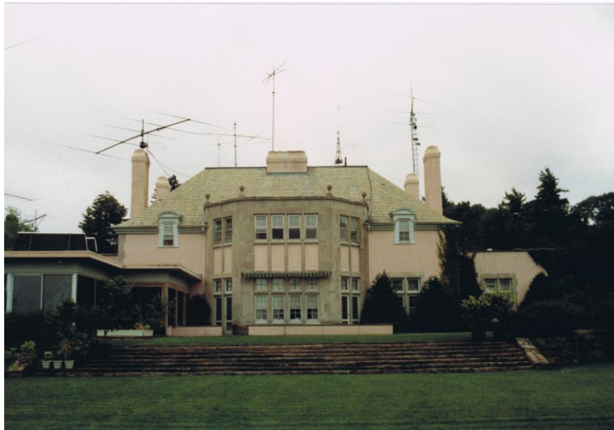
Figure 7-2 - Hazard "Buz" Reeves' house in Tuxedo Park with his vast array of antennas.
