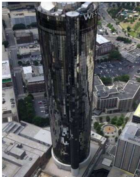
Figure 1.1: Aerial View of the Westin (Image from Skanska)
