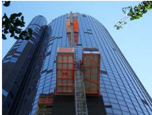
Figure 2.1: Elevator Lifts Used for Window Replacement
