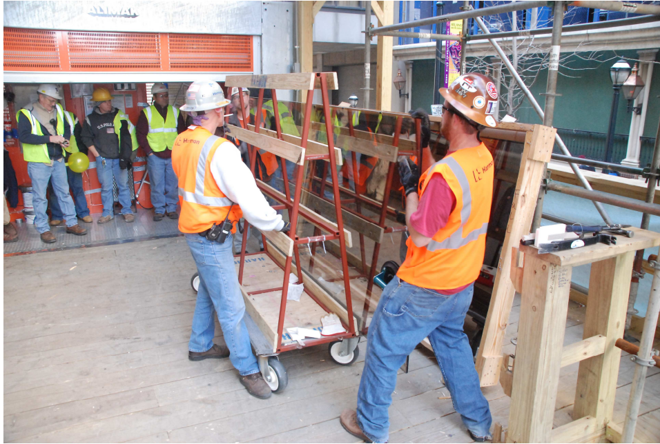
Figure 4.10 Glass from Delivery Truck Placed onto Cart for Transport
