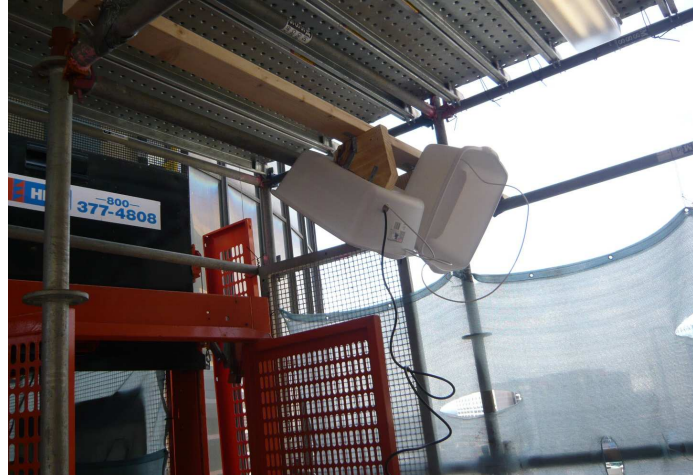
Figure 4.5 Reader and Antenna Placed on Buck Hoist Platform
