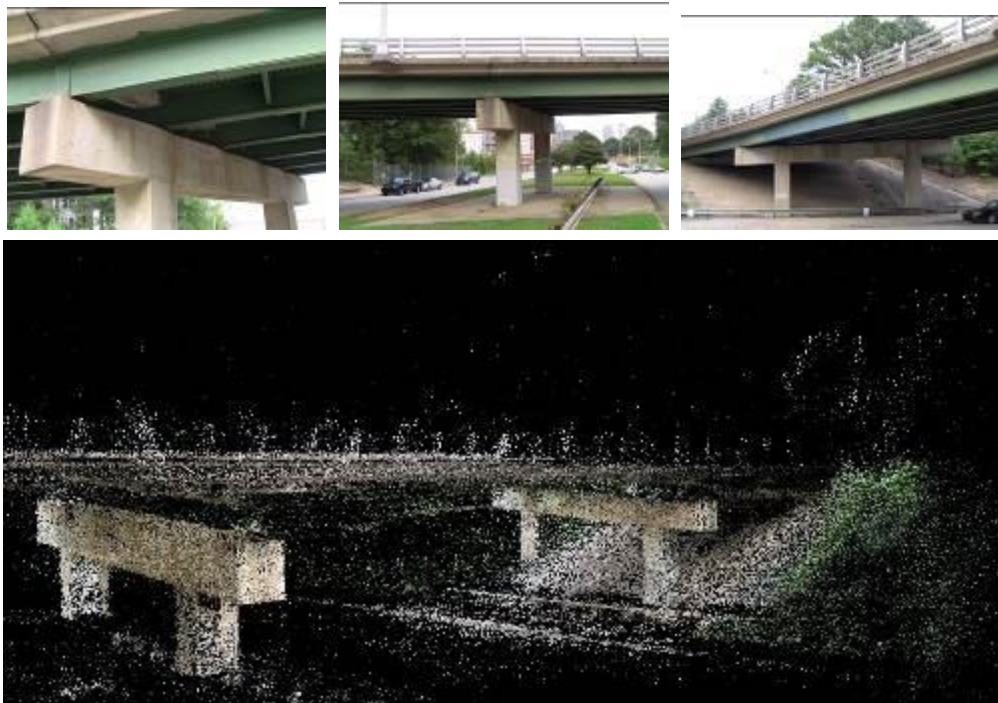
Figure 5.8: Outdoor case study #01: steel bridge with concrete columns
