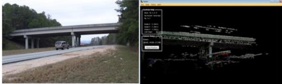
Figure 1.4: 3D point cloud of a concrete column beam bridge
