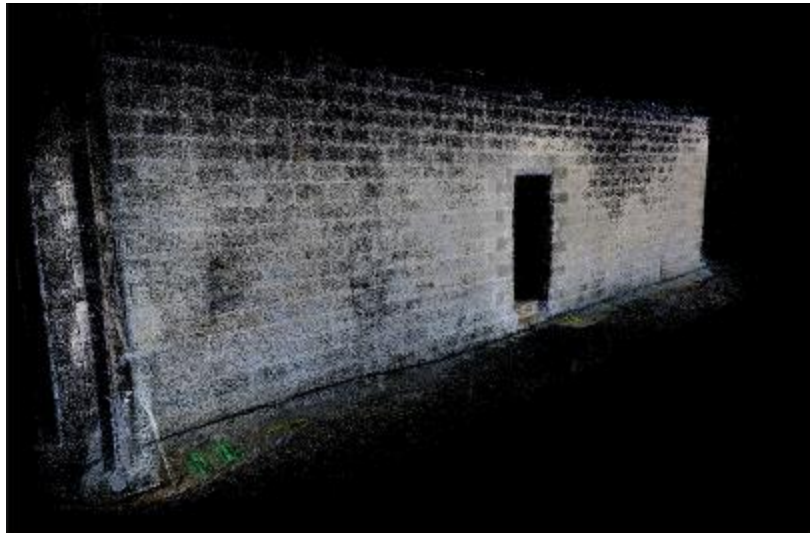
Figure 5.10: Outdoor case study #03: masonry wall in a construction site
