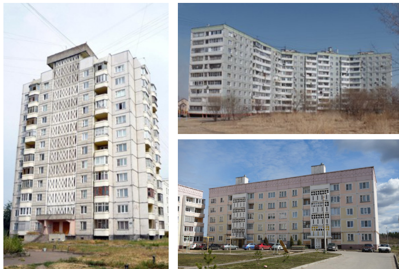
Figure 10: Three examples of Series 121 apartment blocks, demonstrating the typological potential of the series. First: unidentified twelve-story apartment block; second: ten-story curvilinear block for 235 apartments, Tikhookeanskaya Street, Khabarovsk, 1988; third: five-story block, Kislyakov Street, Pskov, 2005. Source: Na dache foto 2015–2021.
