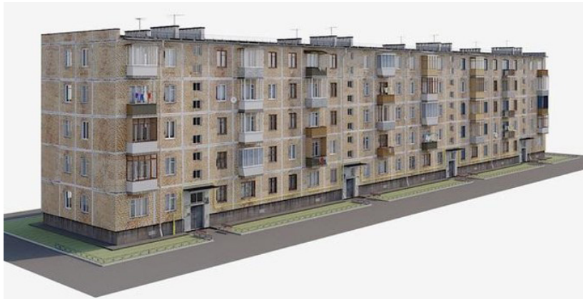
Figure 4: Model of a tile-faced large-panel I-464 block for 80 apartments. Note the mélange of residents' modifications to balconies and windows, disrupting the otherwise homogeneous façade. Source: Putintsev 2019.
