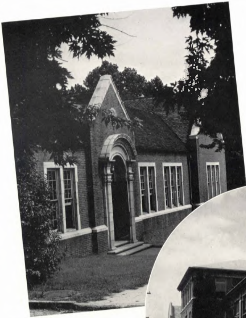
Ceramic Engineering Building
