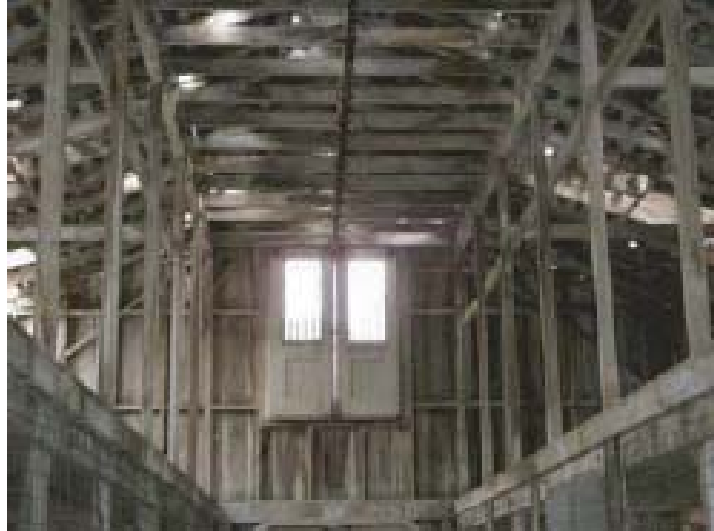
Figure 14 - Interior View of Barn
