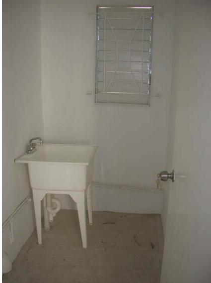
FIGURE 22: TRENCH TOWN Wash Room
