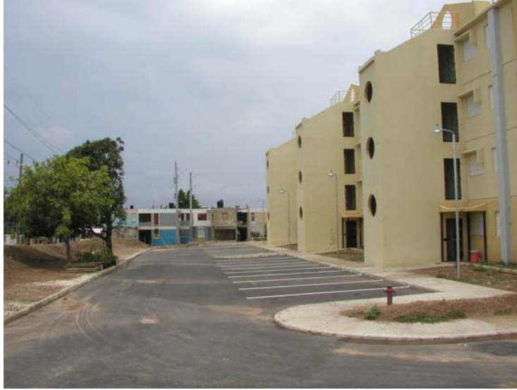
FIGURE 20: TRENCH TOWN Four Storey Housing Units with Enclosed Access Stairwell
