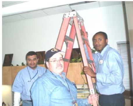
Chuck showing Abe and Andre how to install a motion sensor.
