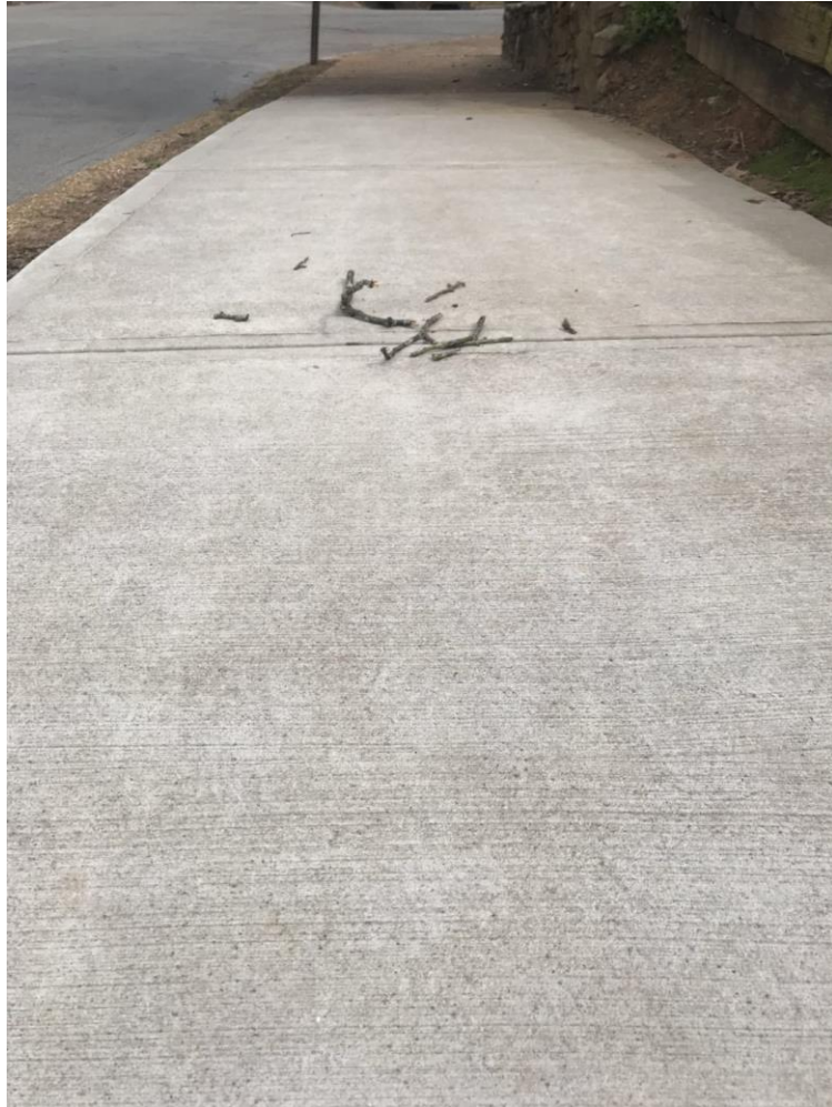
Figure 3. The Concrete Pavement of Control Route.
