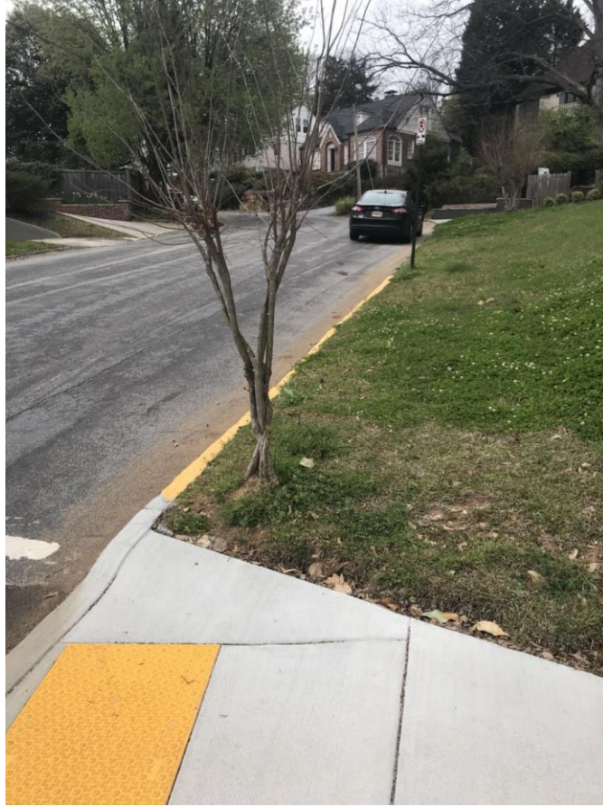
Figure 8. The Missing Sidewalk along the Control Route.
