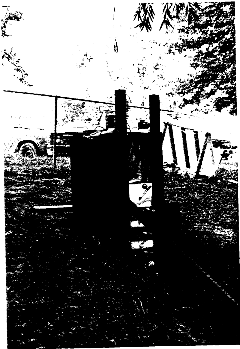
Figure 15 Views of test bed during construction
