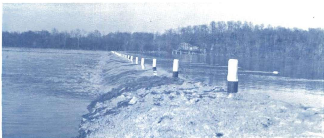
Highway fills across plains coupled with bridges having inadequate openings obstruct flow and increase elevations of flood waters upstream. Effect was more than four feet here during this flood.
