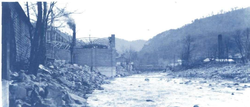
Buildings crowding banks and protruding into the channel reduce capacity of the stream and increase flood heights.
