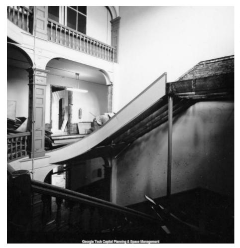
Fig. 3-41: Demolition of main stair, at third floor, 1964. *Georgia Tech Capital Planning and Space Management*.
