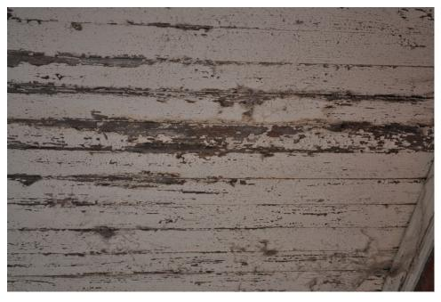
Fig. 3-100: Original tongue and groove ceiling at west entrance porch showing earlier gray paint colors beneath the existing white paint, 2012. *Photo, Beth Grashof.*
