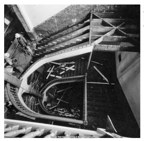
Fig. 3-42: Demolition of main stair, at fourth floor, 1964. *Georgia Tech Capital Planning and Space Management*.
