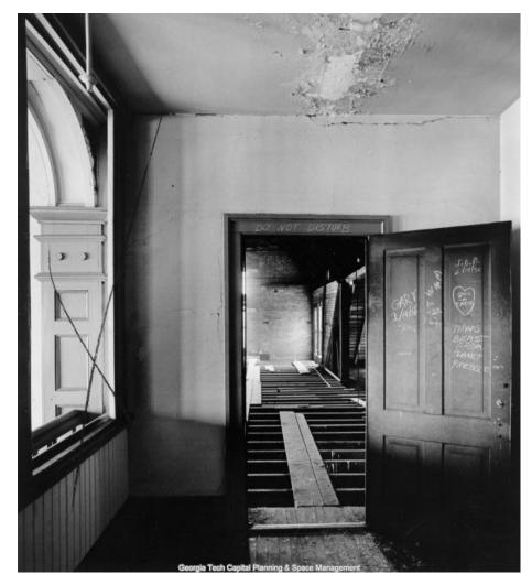
Fig. 3-45: Fourth floor during 1964 interior demolition; looking towards unfinished attic at east end of building. Georgia Tech Capital Planning and Space Management.
