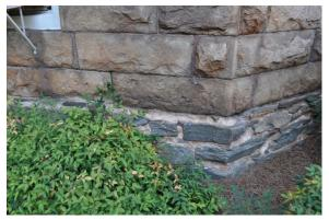
Photo #24 – Detail showing rubble foundation wall and rock-face ground floor walls; east elevation.
