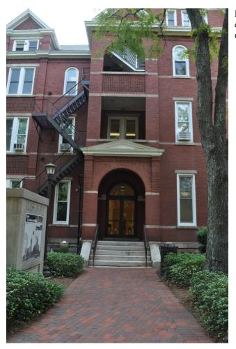
Fig. 3-99: Partial west elevation showing west entrance porch and one of several fire-escapes in existence since at least 1948.
