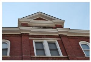
Photo #25 – Detail of cornice at third floor and fourth floor dormer, east elevation.
