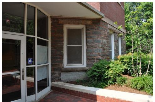
Fig. 3-112: North basement entrance at point where water closet was once located; note window at basement chapel bay which was once a door into the College Inn; 2011. Photo, Beth Grashof.
