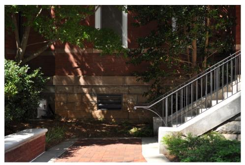
Fig. 3-93: Detail, front entrance porch showing later handrail of compatible design that meets handicapped accessibility codes, 2011. *Photo, Beth Grashof.*
