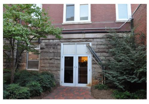
Fig. 3-120: Detail of northeast basement entry in former window opening; appears to have been done prior to 1960s renovations; 2011. *Photo, Beth Grashof.*
