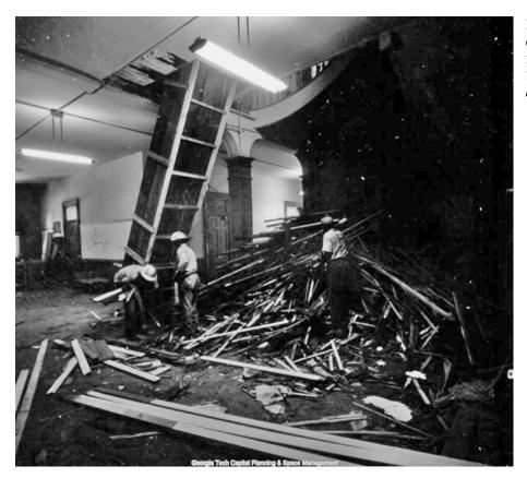
Fig. 3-40: Demolition of main stair, at first floor, 1964. *Georgia Tech Capital Planning and Space Management.*
