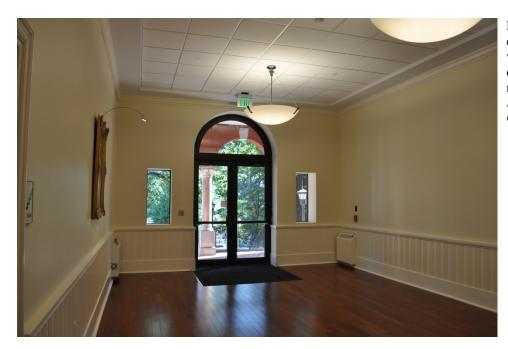
Fig. 3-123: Main entrance vestibule; wainscot installed during 2010 renovation; 2011. Photo, Beth Grashof.
