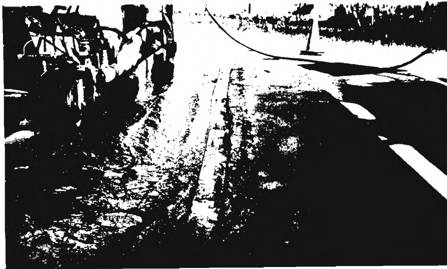
a. Cutting Groove in OGAFC
