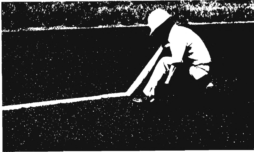
e. Removal of Masking Tape Used for Surface Protection
