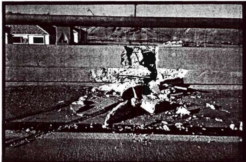
Figure 18 - Pounding Damage due to the 1994 Northridge Earthquake.
