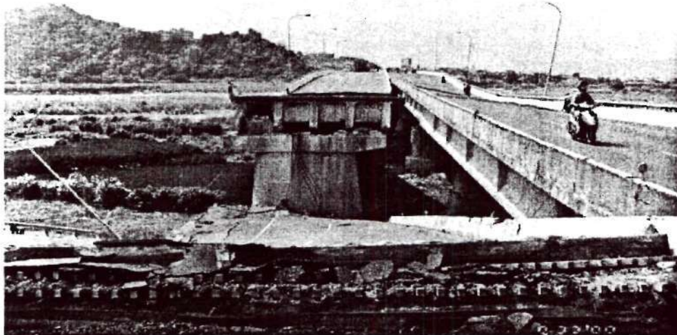
Figure 24 - Span Unseating due to the 1999 Taiwan Earthquake.
