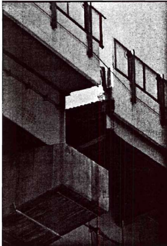
Figure 22 - Permanent Hinge Opening due to the 1995 Kobe Earthquake.
