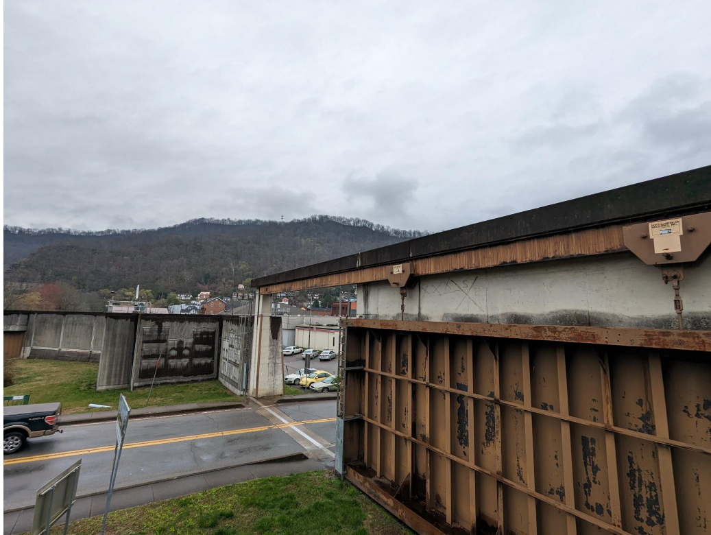
Figure 9. Flood gate for Williamson, West Virginia along the Tug Fork River (Photo by author 2023).
