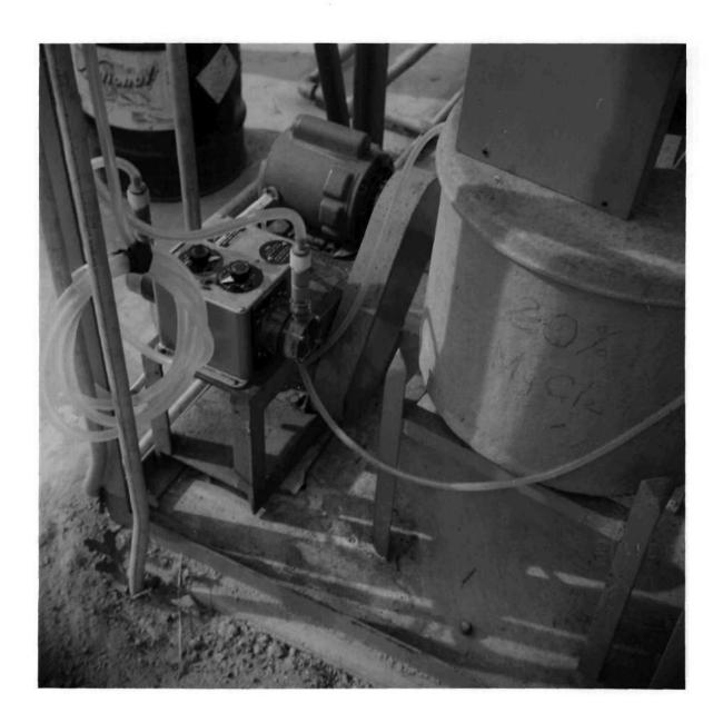
Figure 8. Picture of the Dual Chemical Feed Pump
