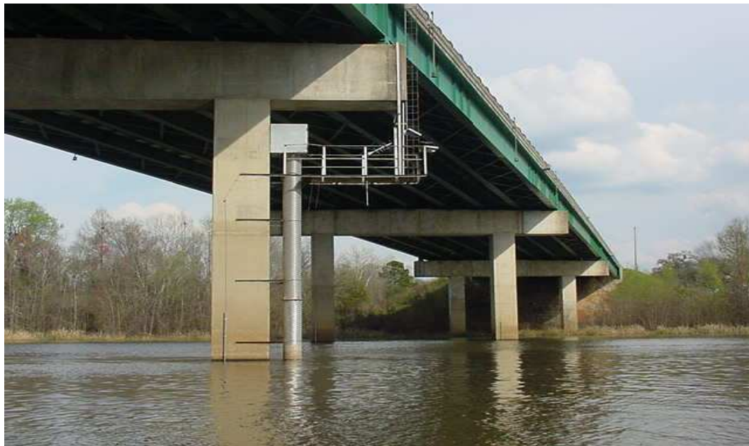
Figure 3.8 Bridge pier bents in Flint River at Bainbridge, GA
