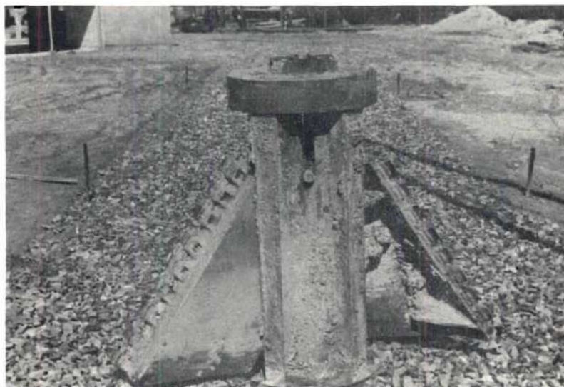
Fig. 3. Reaming Bit
