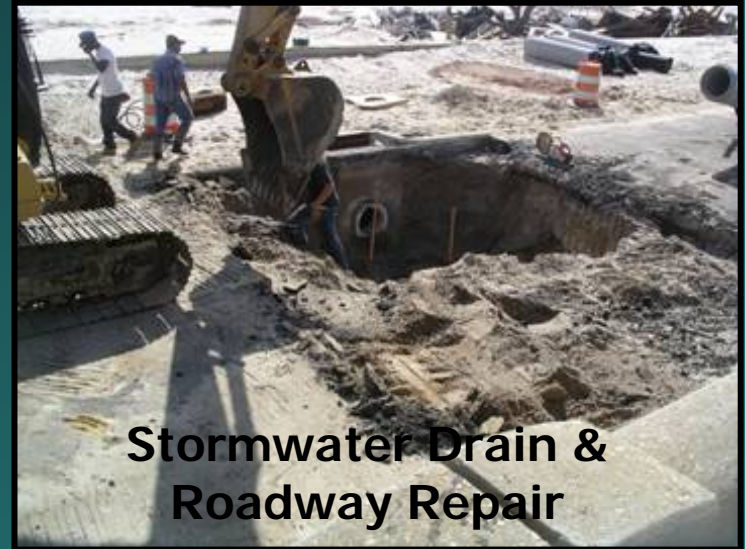
Box Culvert Replacement
