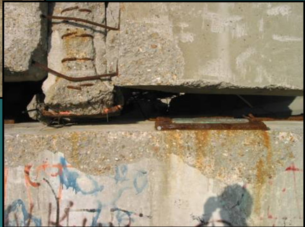
Steel-Bronze Bearing Damage
