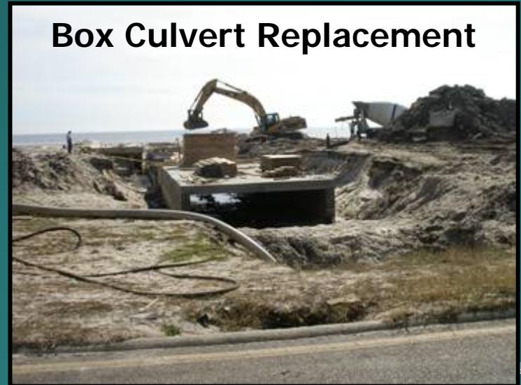
Stormwater Drain & Roadway Repair
