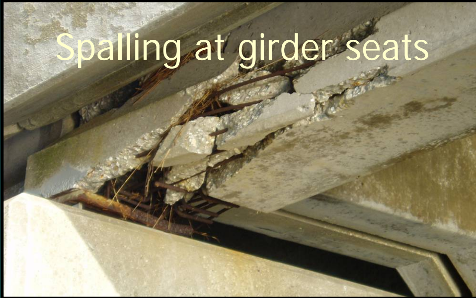
Spalling at bent caps
