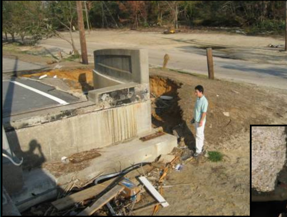
Abutment Damage and Loss of Backfill
