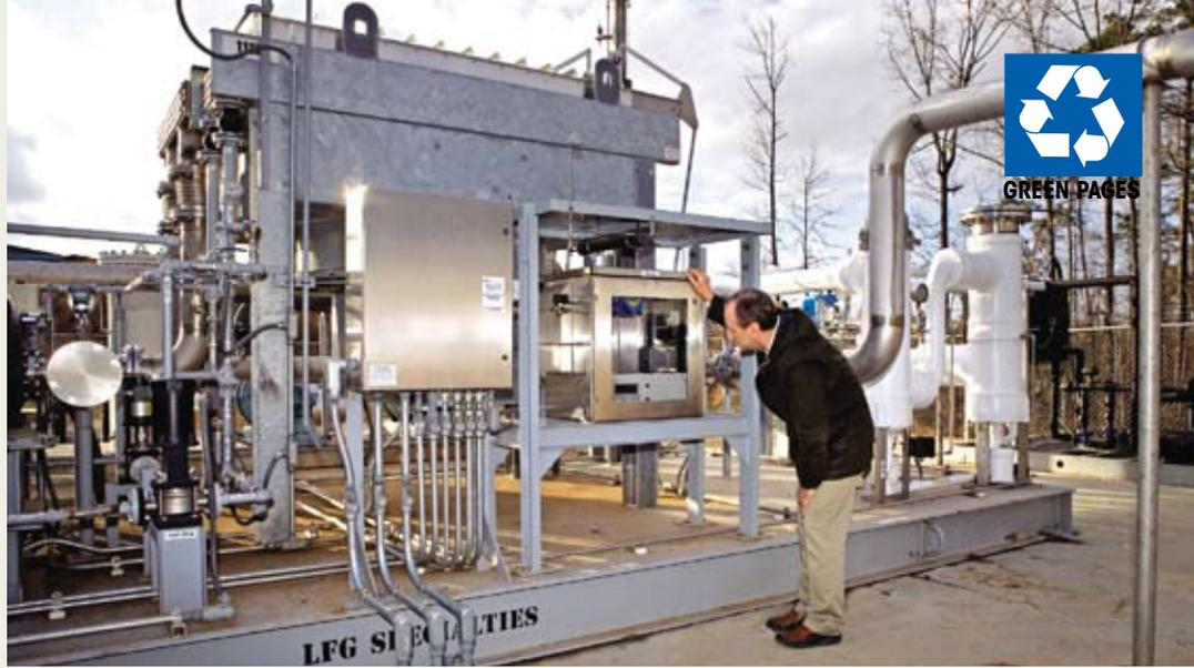
*Interface Inc. pipes in methane gas from a nearby landfill in LaGrange, Georgia, to power one of its plant processes. Here VP of Engineering, David Gustashaw, monitors the gas analyzer. As methane is drawn off to fuel the factory, the entire landfill volume is drawn down, increasing its capacity and postponing the city's next landfill opening for an estimated fifteen years.*
