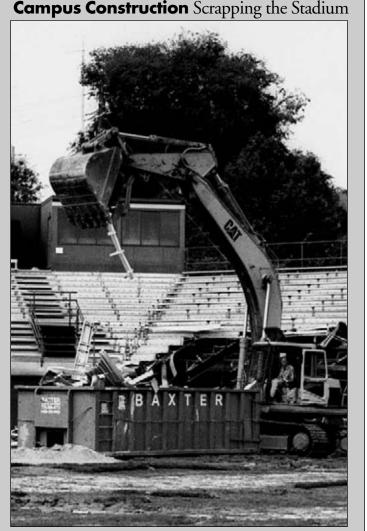
By Bill Allen / STUDENT PUBLICATIONS The bleaches of Russ Chandler Stadium are torn down by a front end loader. The destruction is part of renovation plans designed to increase the seating capacity of the stadium.
