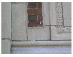
Figure 106: The pointing mortar used in this stone repair at D. M Smith does not appear to match the historic mortar.
