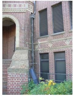
Figure 104: Biological growth and mortar deterioration associated with the location of a downspout on the O'Keefe Main Building.
