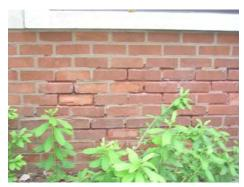
Figure 105: Image of significant mortar deterioration and brick spalling along the base of a historic building.
