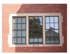
Figure 103: The character of the original multipane windows was replicated in the replacement units installed during the recent rehabilitation of the Old Civil Engineering Building.
