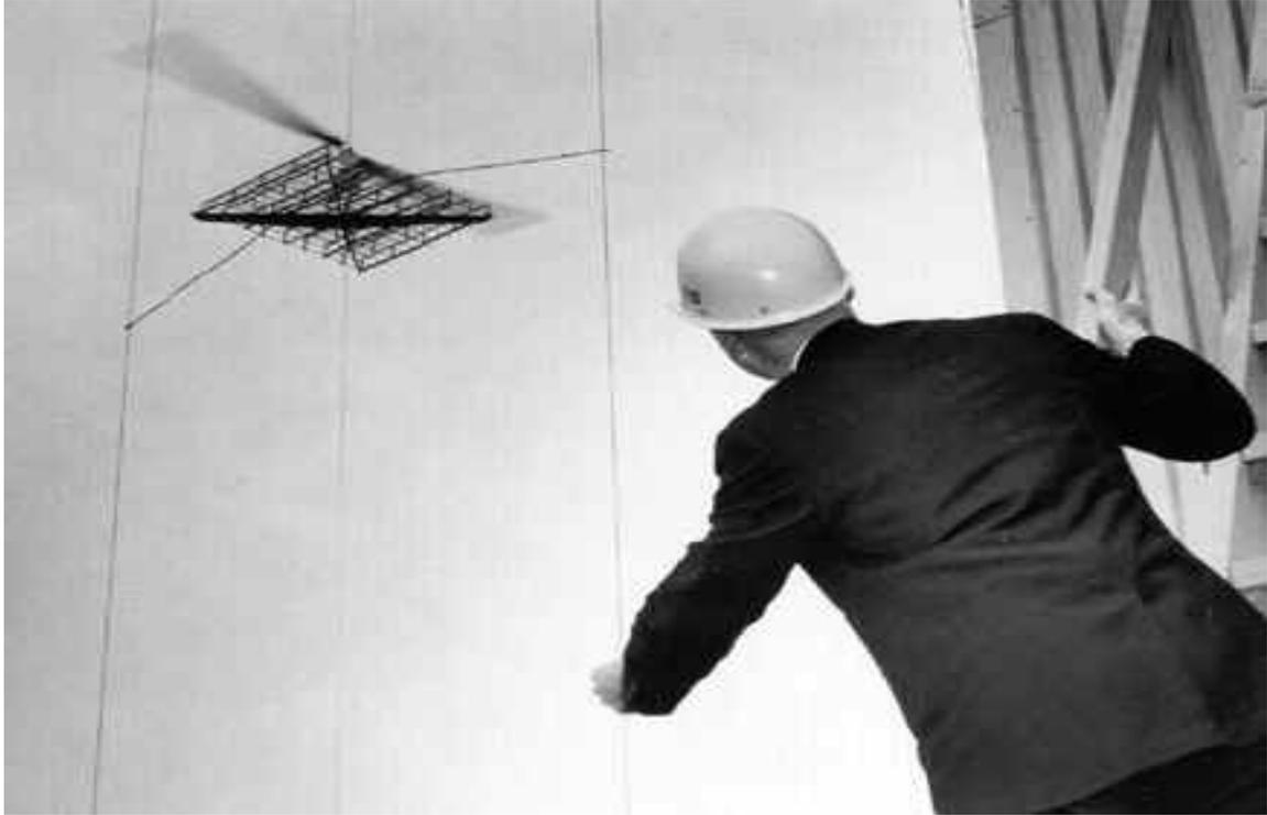
**Figure 2.3:** Demonstration of the rectenna helicopter on Oct 1964
