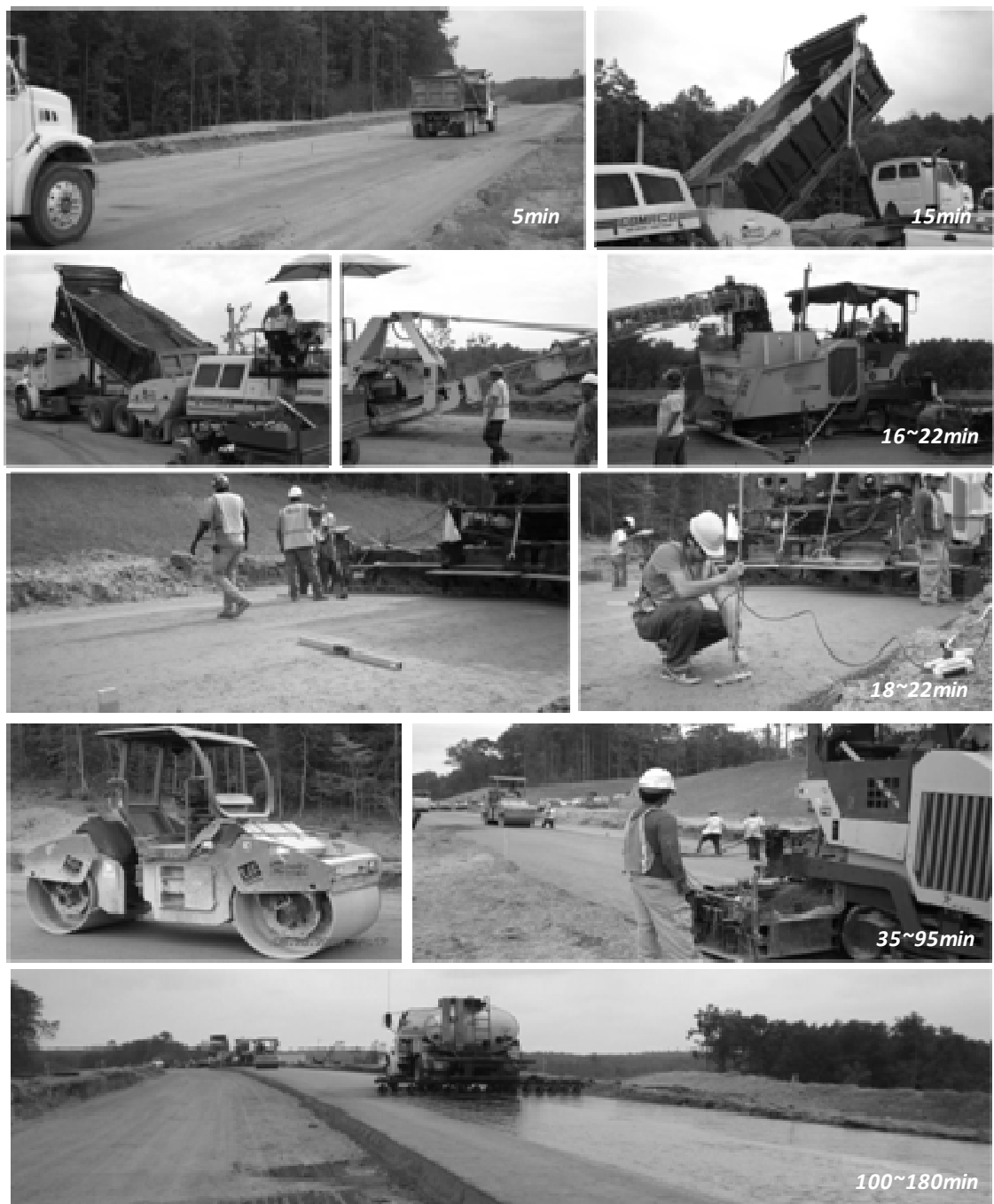
Figure 2.4 Cement-treated base construction monitoring from the time water is added to the mix to the final bituminous cover.
