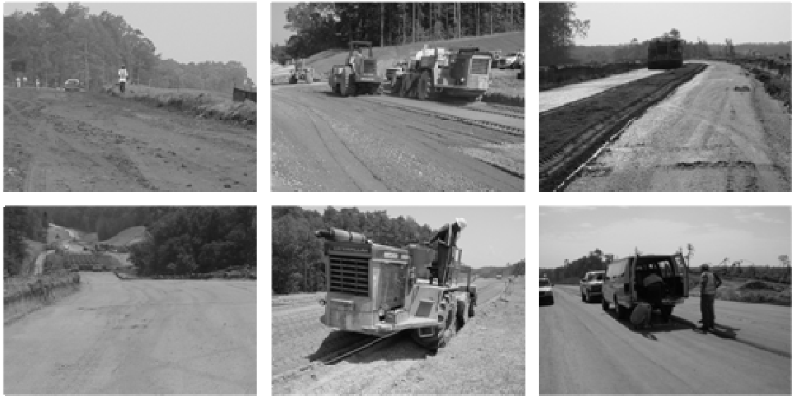
Figure 2.3 Stabilization of the subgrade upper 0.15m through addition of unbound aggregate base and re-compaction.
