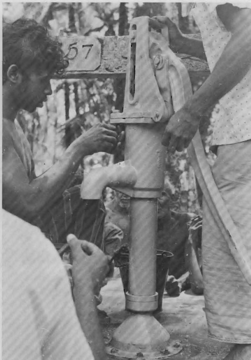
Figure 27. Bolting Cap Assembly onto Pump Body
