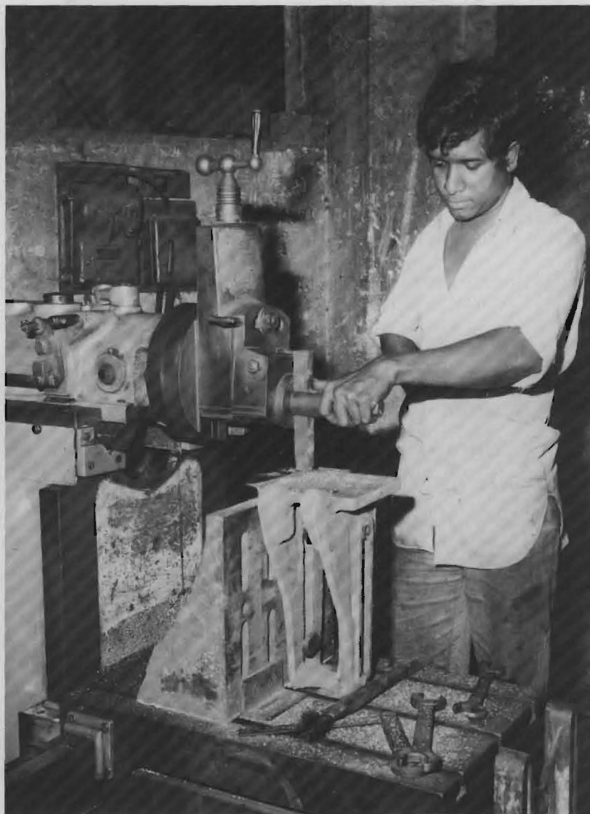
Figure 11. Machining the Pump Cap
