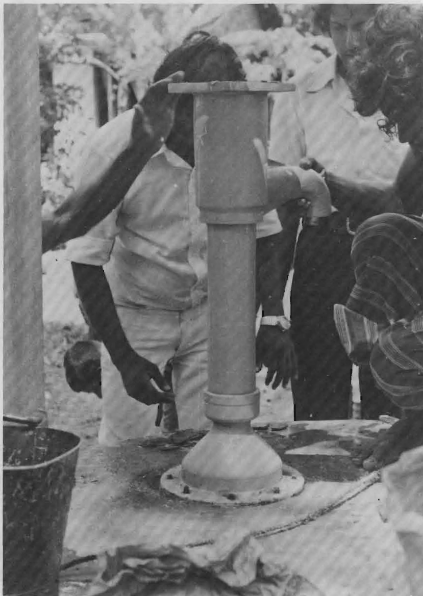
Figure 26. Bolting Pump Body and Base to Well Cover
