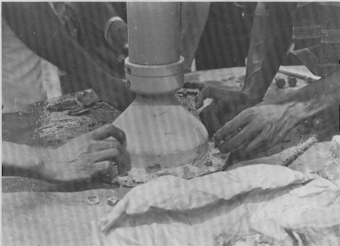
Figure 20. Securing the Pump to the Concrete Cover Platform
