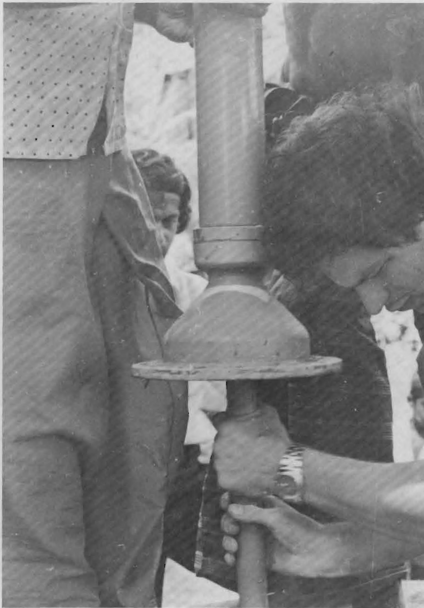
Figure 19. Attaching the Drop Pipe to a Shallow-Well Pump
