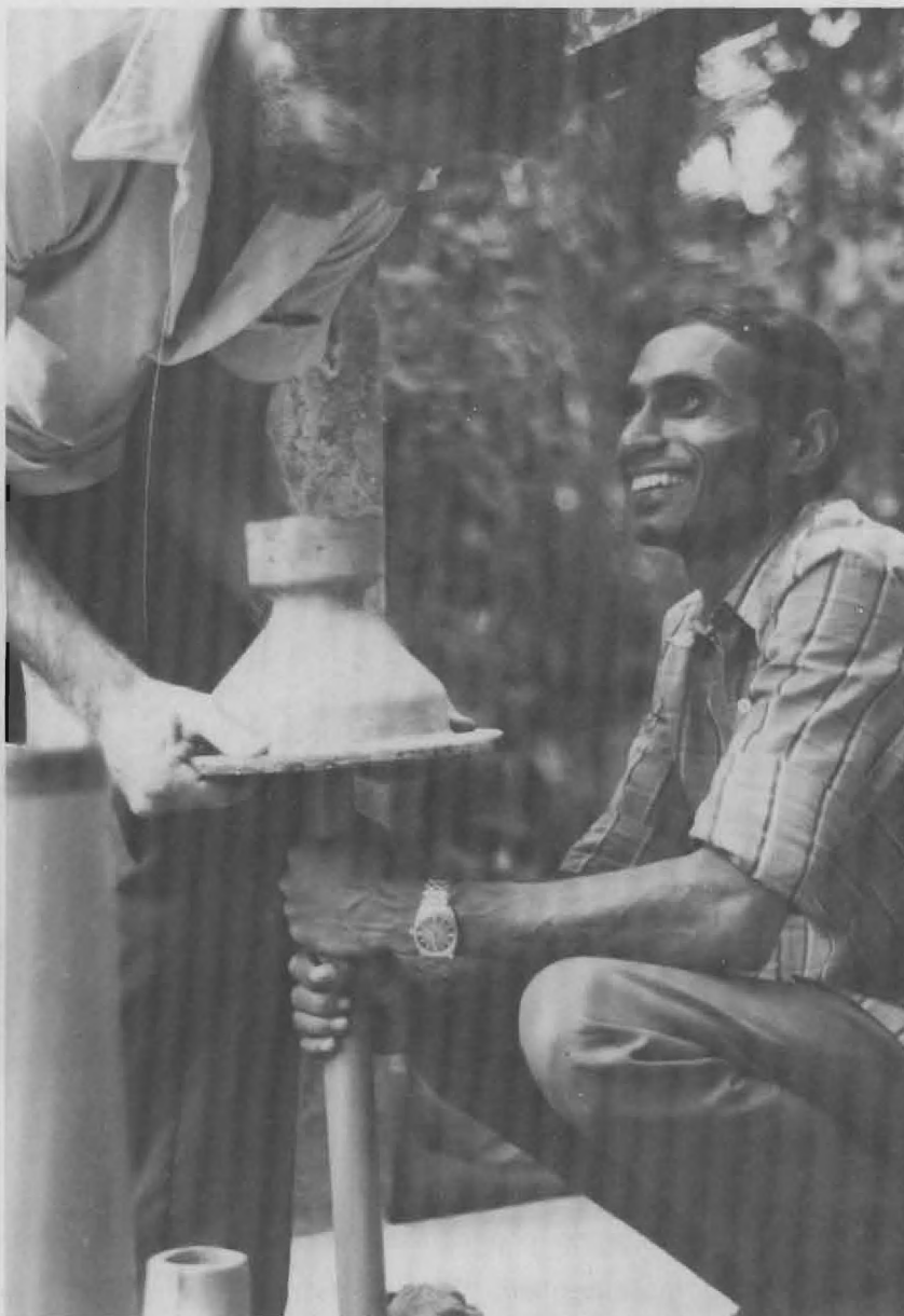
Figure 25. Attaching Drop Pipe to Pump Base
