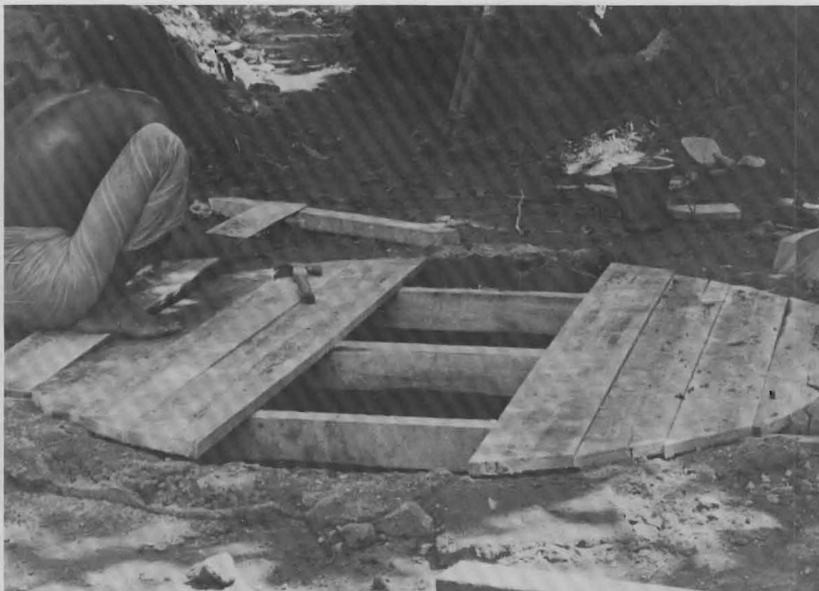
Figure 14. Construction of Formwork
