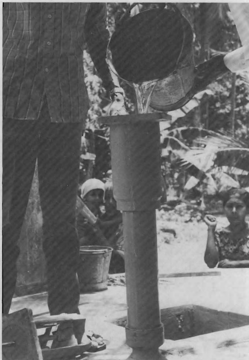
Figure 21. Initial Priming of the Pump
