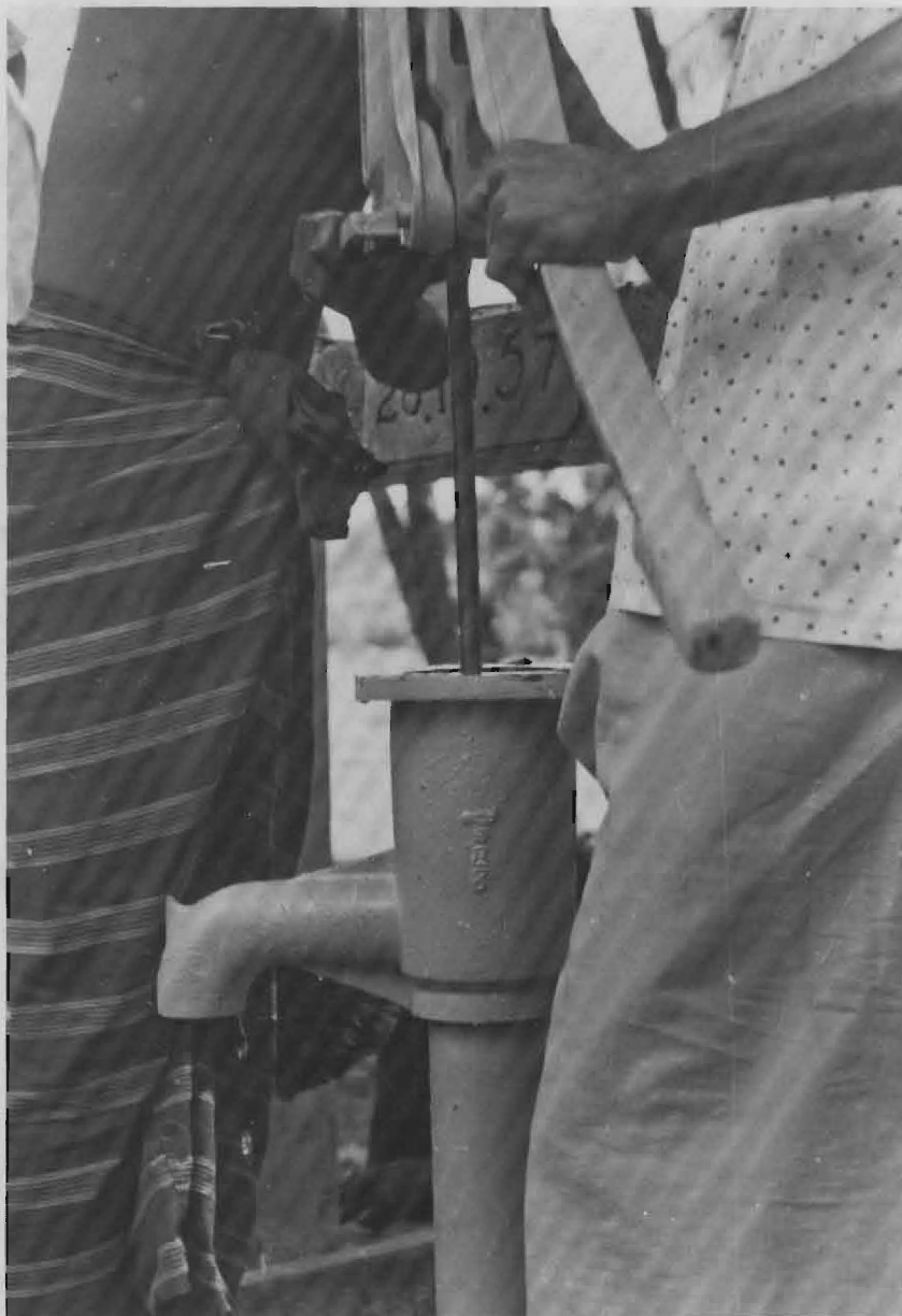
Figure 22. Lowering the Cap onto the Pump
