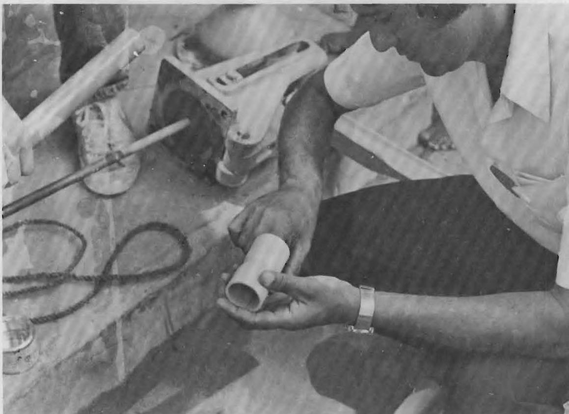
Figure 24. Assembly of PVC Drop Pipe
