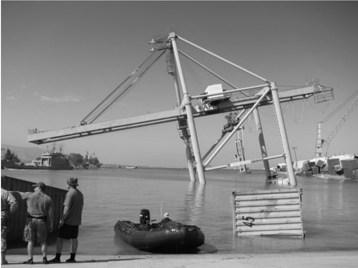
Figure 1.2: Partially submerged container crane at the port in Port-au-Prince following the January 12, 2010 earthquake (Photo courtesy of Glenn Rix)
