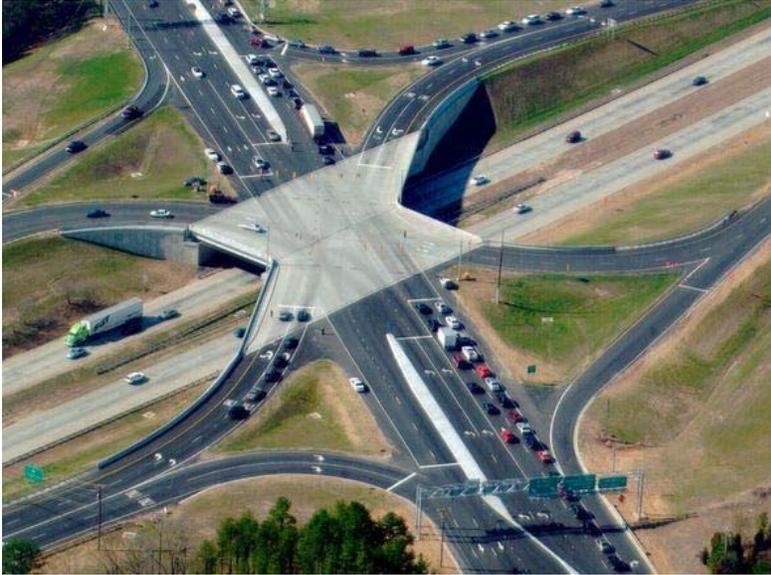
Figure 32. Example of SPUI form from I-40 in Durham, NC
