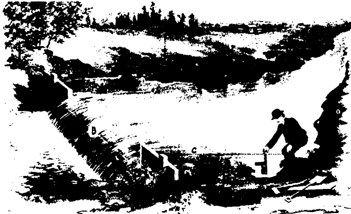
Measuring Flow of Water by Weir Method
