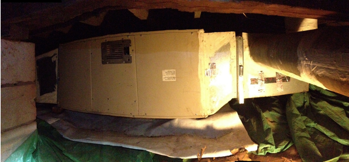
Figure 15 Test system 1 is located in an unconditioned crawlspace and is horizontally configured. The return plenum is on the right and supply plenum to the left.
