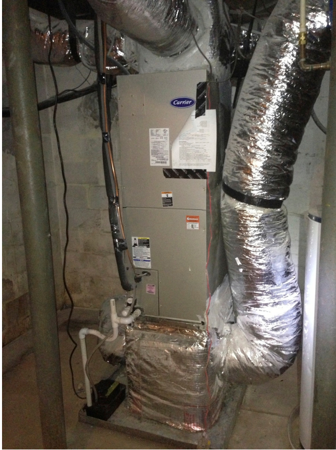
Figure 16 Test system 2 is vertically configured and located in an unconditioned basement. The return plenum is on the bottom and supply plenum above.
