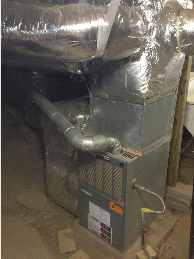
Figure 17 Test system 4 is vertically configured and located in an unconditioned basement. The return plenum is on the left side and supply plenum above.
