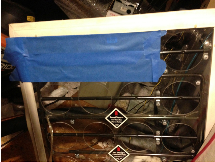
Figure 8 An example of a partially taped filter (“TrueFlow Taped 1”)
