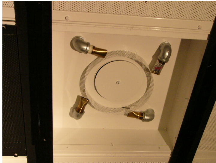
Figure 2.6: Arrangement of Fog Nozzles Inside ORS Diffuser
