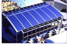
The Georgia Tech Aquatic Center's roof holds a 342kilowatt photovoltaic (PV) system, which will provide significant, long-term data on how to build and maintain large-scale PV structures. (200-dpi JPEG version - 362k)
