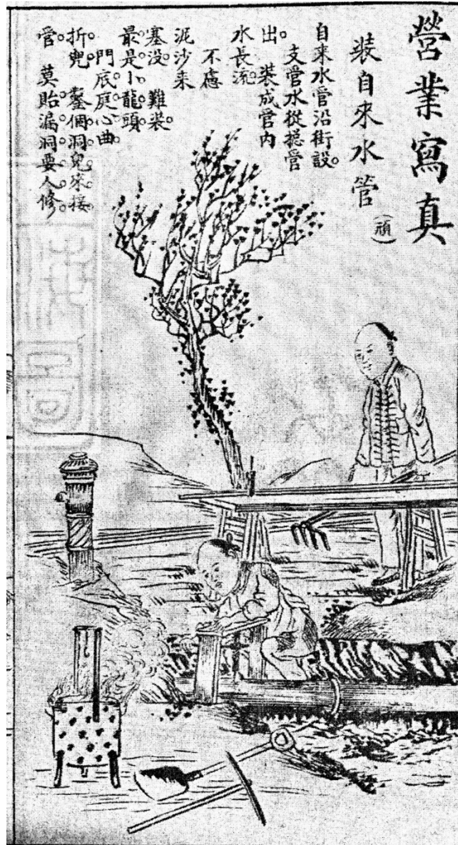
Figure 5 – Chinese coolies laying water pipes. A hydrant can be seen on the left side. Source: Wan, 1910.
