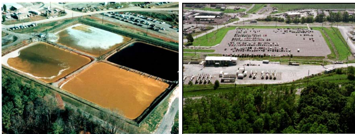
Figure 1.1 The former S-3 Waste Disposal Ponds located near the Oak Ridge Y-12 Plant in Bear Creek Valley (left). The unlined ponds received highly acidic uranium nitrate liquid wastes from 1951 to 1983 (Brooks, 2001). The ponds were capped in 1984 after treatment and removal of liquid wastes (right). Picture from http://public.ornl.gov/orifc/orfrc3_site.cfm#Anchor1 .
