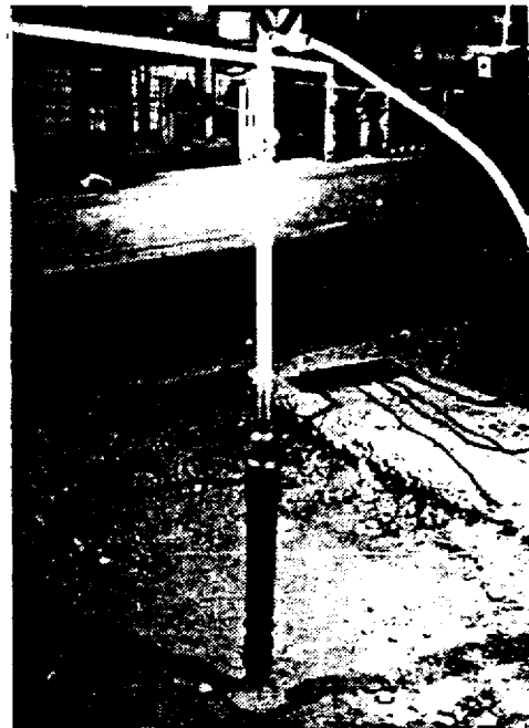
Figure D-6. Single Legged Pneumatic Compactor Used on Subgrade.
