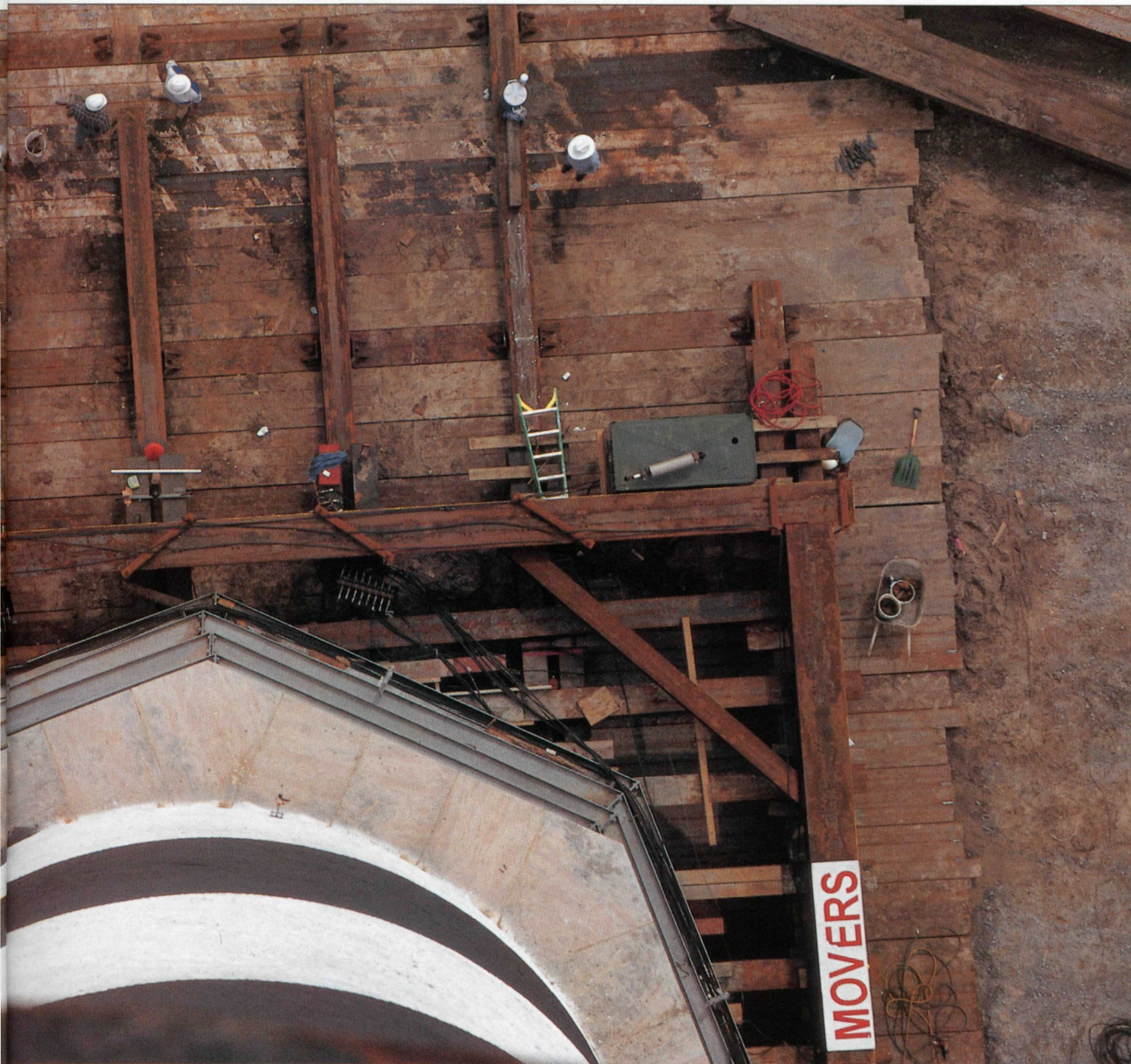
The 70-foot-long guide rails are laid on 190-foot-long steel mats, which lie on a 700-foot-long section of compacted gravel.
