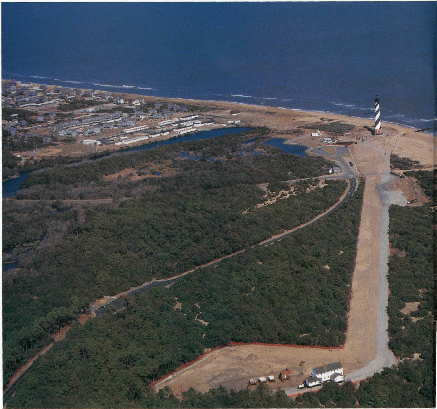
The 2,900-foot-long move corridor awaits the lighthouse's transfer to the new site, about two feet higher than the old.
