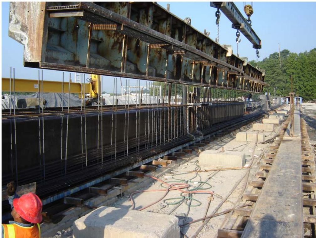
Figure 4.7 Straddle-lift placing form around reinforcing bars
