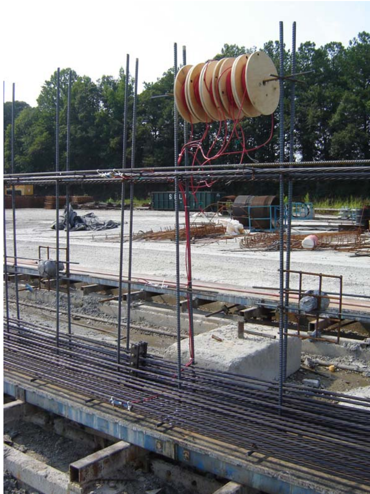
Figure 4.6 VWSG locations and wire secured above girder
