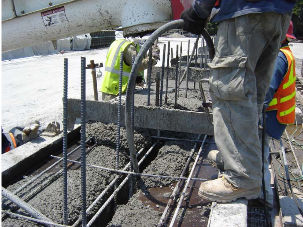
Figure 4.14 Workers vibrating concrete in the web of the girder
