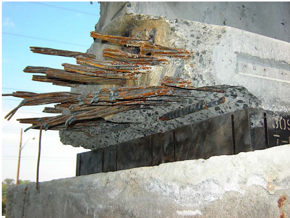
Figure 8.5 Girder end resting on elastomeric bearing pads; Friction between the beam and the construction bed during prestress strand cut-down caused the friction failure shown here, which was corrected in the field.
