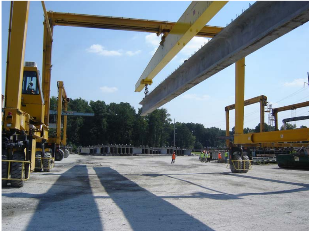
Figure 4.20 Straddle lift moves through the yard to store girder
