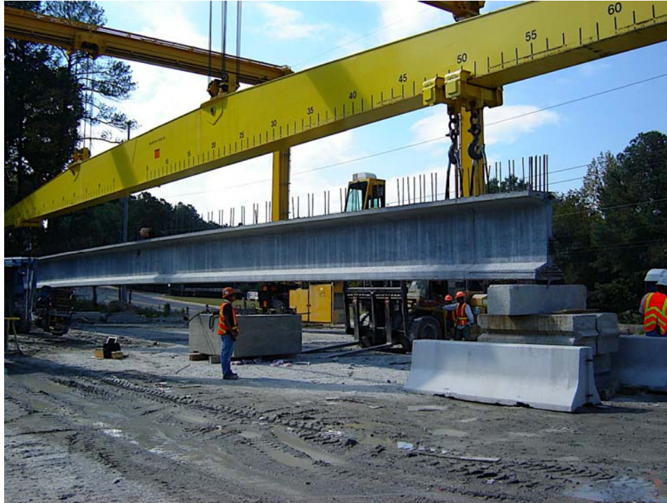
Figure 8.4 Crane setting girder on dunnage supports
