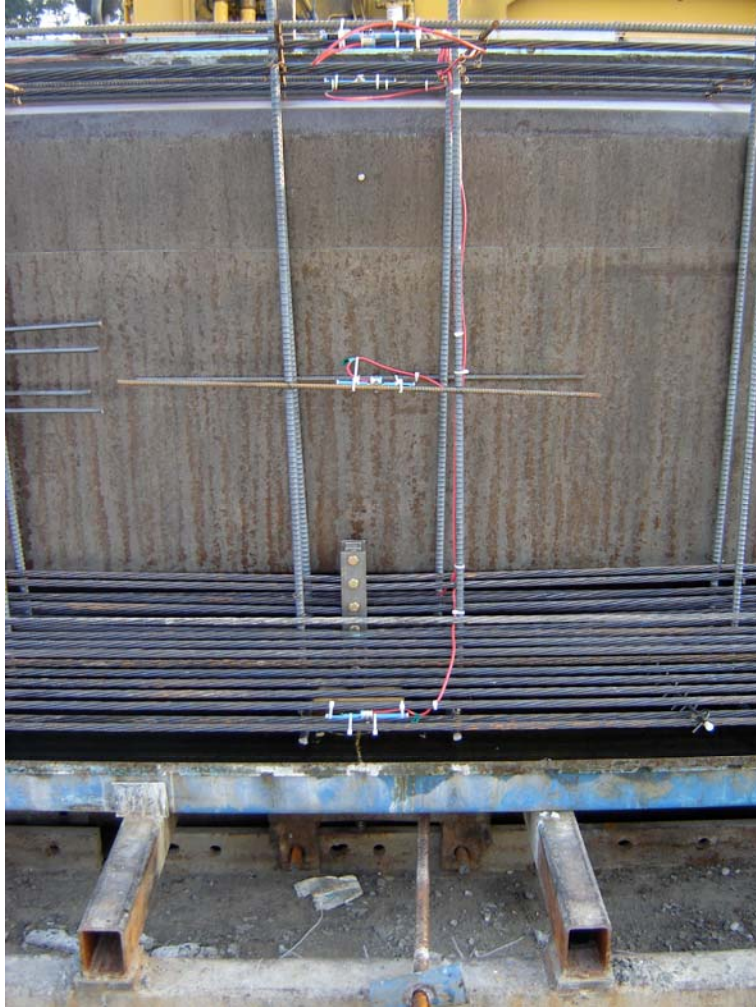
Figure 3.5 VWSG secured with one side of forms placed
