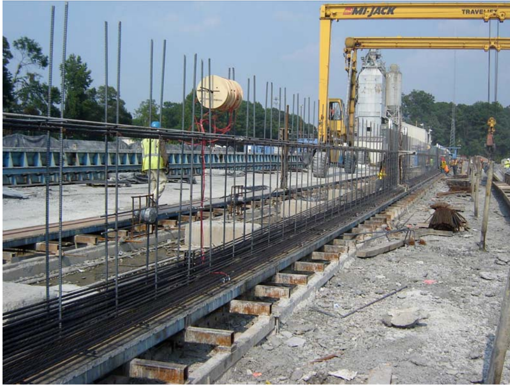
Figure 4.4 Reinforcing bars across 2 girders
