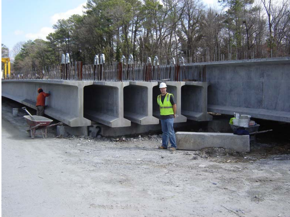
Figure 4.21 Girders stored together in SCP yard
