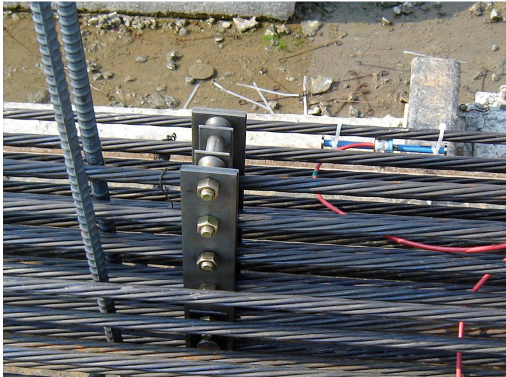
Figure 8.3 Strand harping device detail
