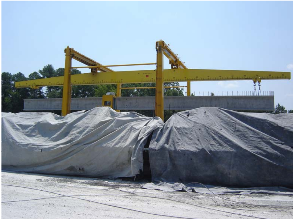
Figure 4.15 Tarps cover the girders to aid in curing
