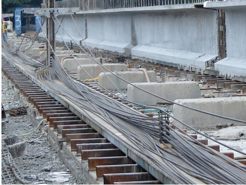
Figure 8.2 Strand harping device being held down to construction bed by a threaded rod
