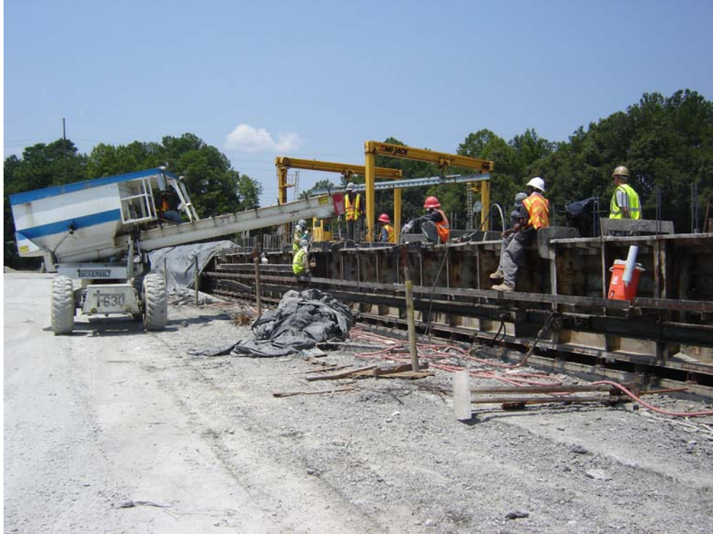
Figure 4.12 Tuckerbilt delivering concrete to forms
