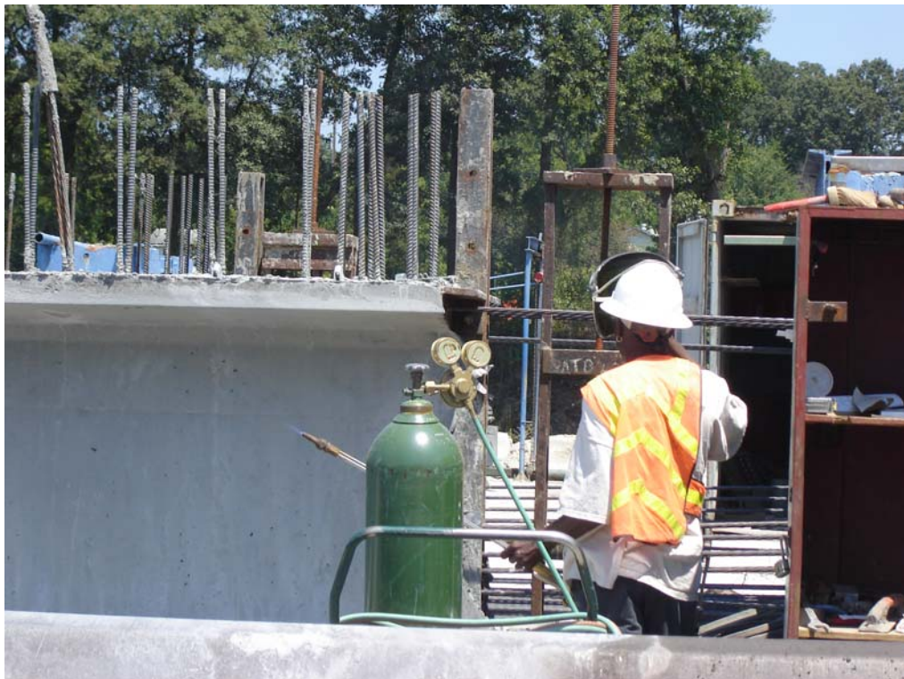
Figure 4.17 Lead worker examines next strand to be cut
