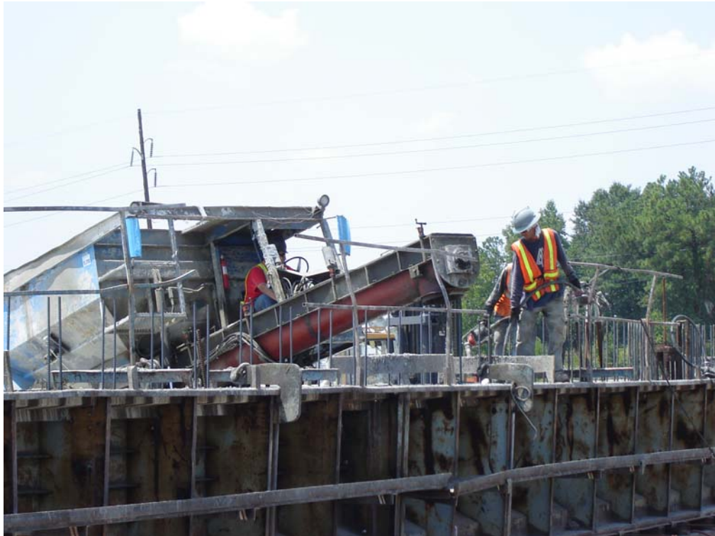
Figure 4.13 Tuckerbilt placing concrete into forms with worker using vibrator
