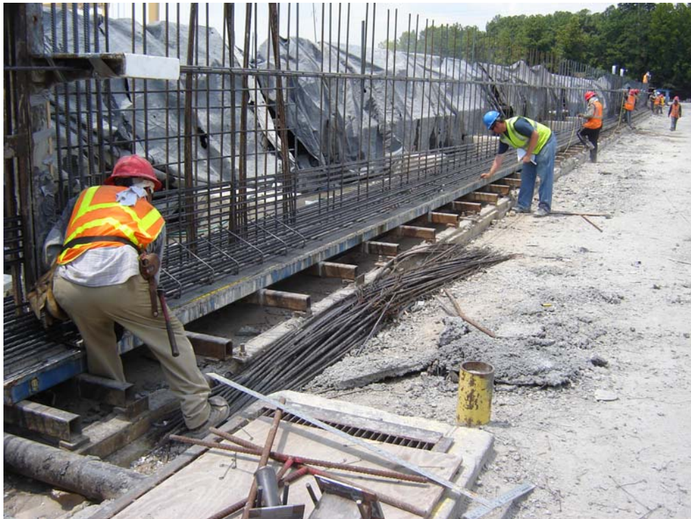
Figure 4.5 Quality Control checking reinforcing bar placement
