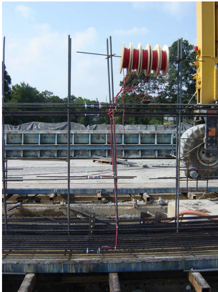
Figure 3.4 Gages in place with wires running up to bundled spools of wires above
