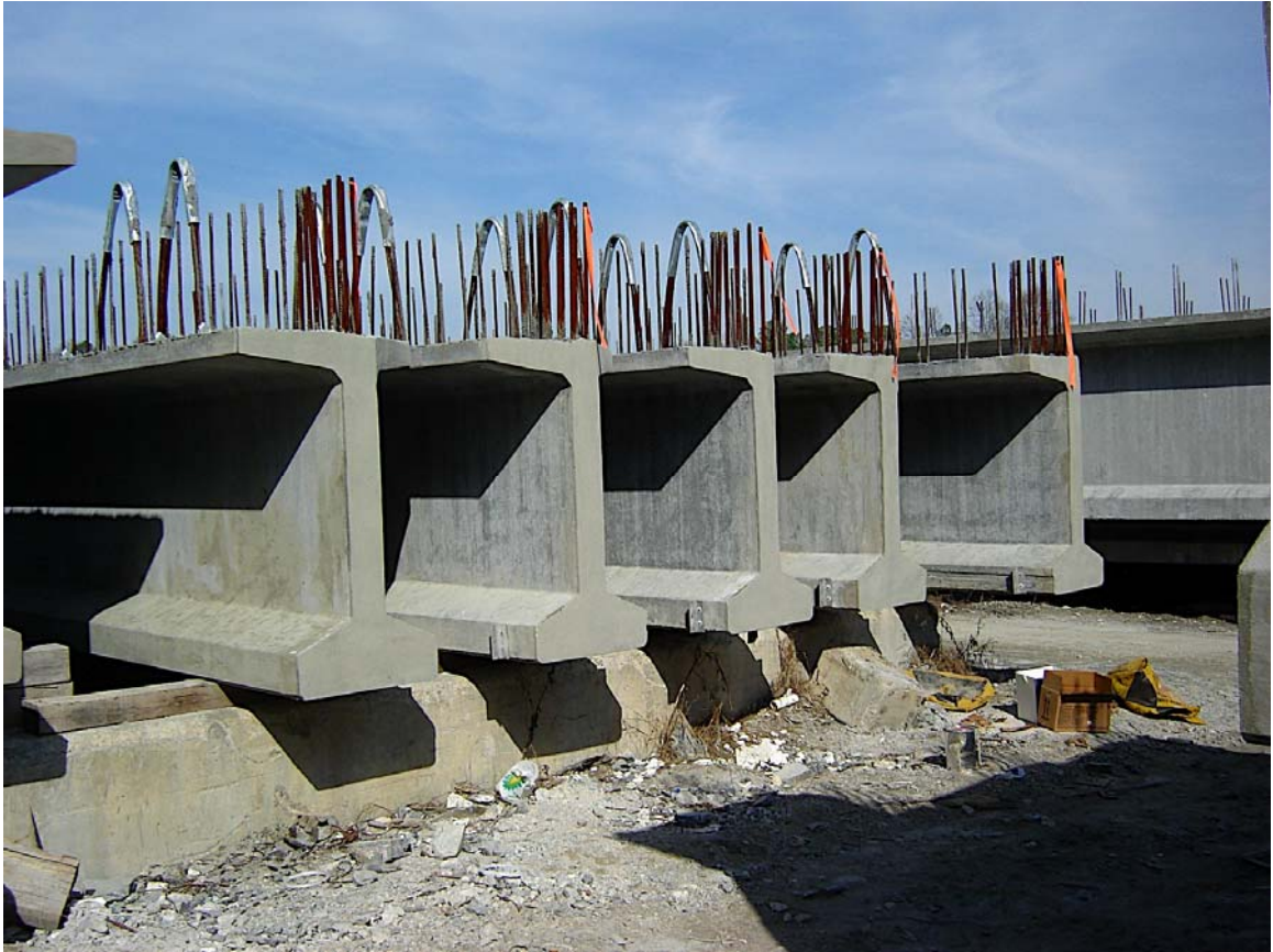
Figure 7.2 South ends of girders set at varying lengths from the end
