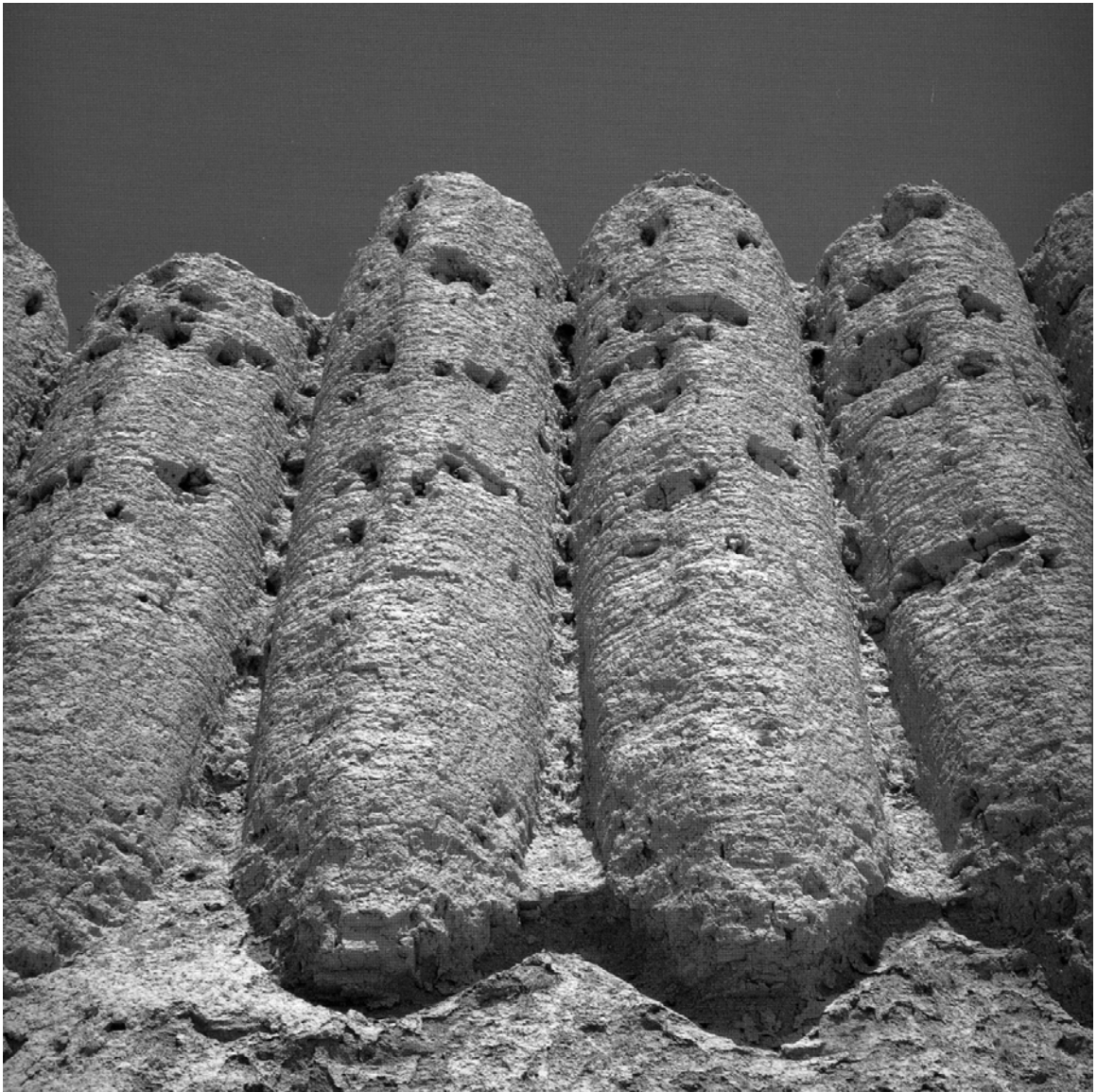
Figure 56: The defensive walls of the city of Merv, still-surviving in certain areas. All of these walls were made of adobe, constantly maintained over the centuries, and were in several instances rose between 10 - 20 meters above the surrounding landscape.
