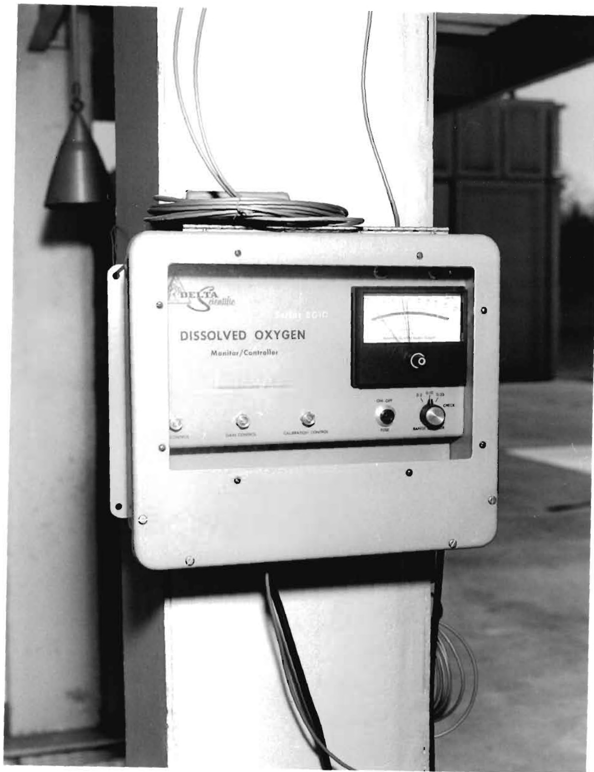
Figure 9. Dissolved Oxygen Analyzer/Controller of Delta Scientific installed at Flint River Plant, Atlanta, Georgia.
