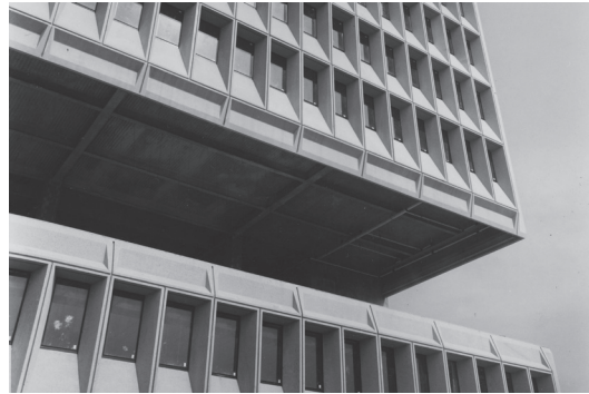
Figure 8: Exterior view of the sandblasted concrete façade with scoring next to the outer edge. Armstrong Rubber company building, 1968-70. ( Ben Schnall, Syracuse University Library 1965-1969)
