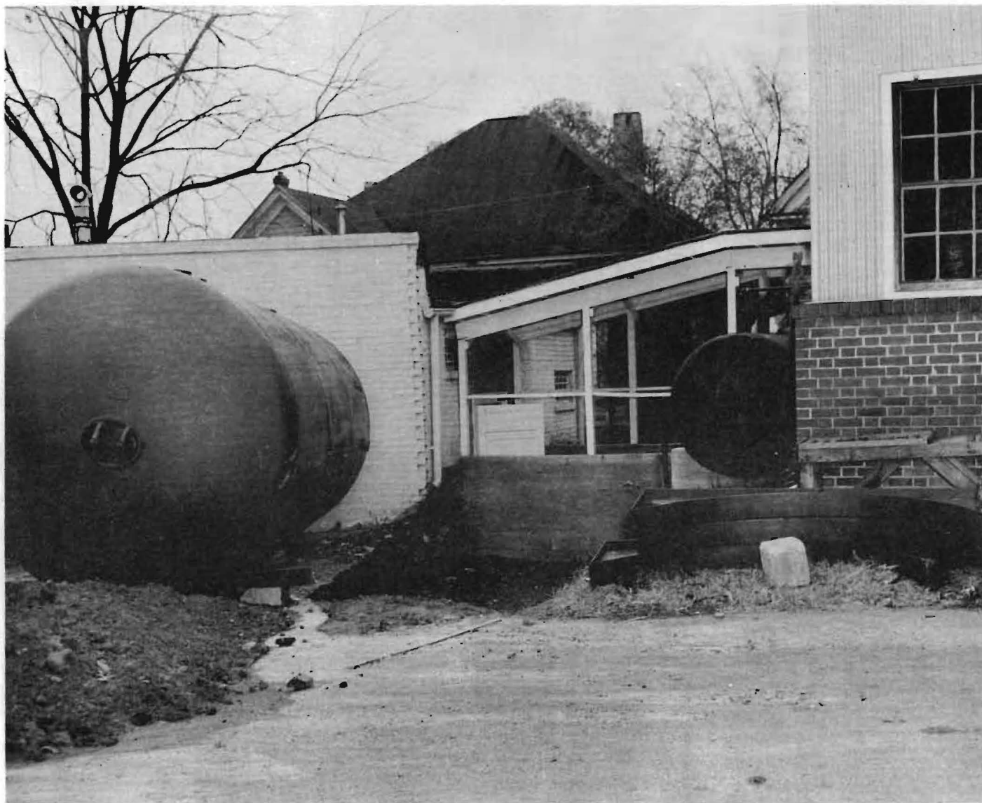
Figure 3. 1000 Cubic Foot Reservoir and Excavation.
