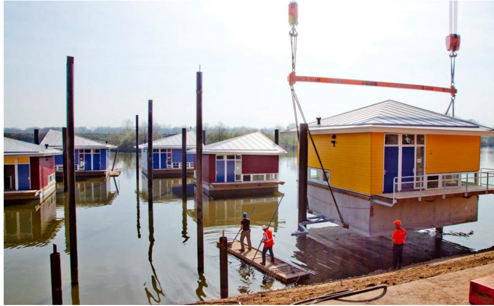
Figure 5.12 ( home being placed on piers by crane ) ( http://www.maasvilla.nl/villas )
