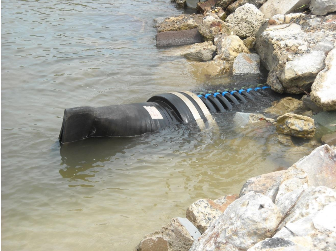
Figure 3.3 ( Backflow Preventer Retrofit preventing backflow on Tybee Island )
