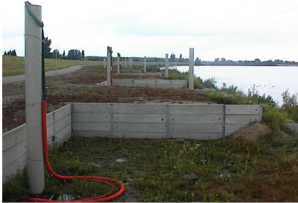
Figure 5.1 (mooring poles between the caissons of 2 neighboring homes) ( boiten.net/watervillas-gouden-kust-maasbommel/ )
