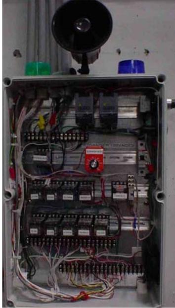
**Figure 12: Main Box for Relays/Controls for Safety System**
