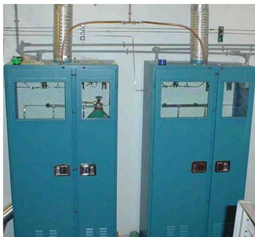
**Figure 5: Gas Storage Cabinets for Hydrogen and Carbon Monoxide Gas**
