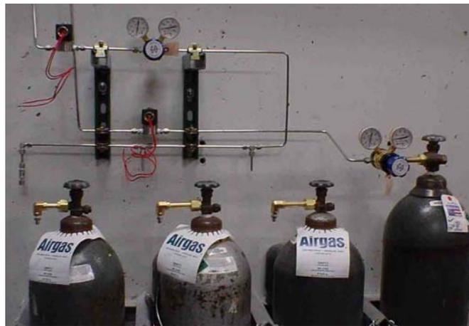
**Figure 8: Bottle Valving and Controls for Carbon Dioxide (Left) and Nitrogen (Right)**
