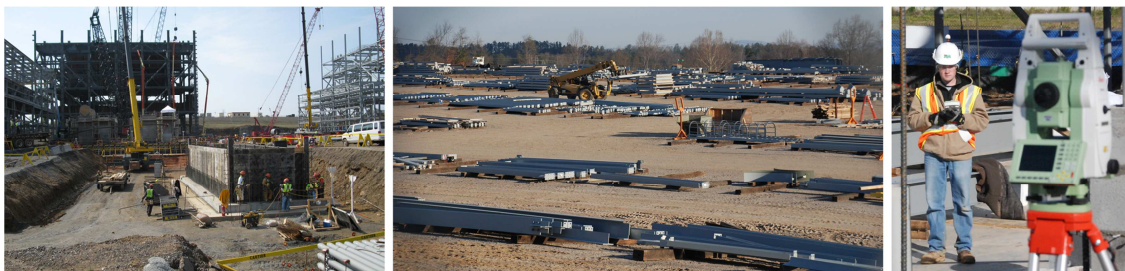
Figure 10 Layout of experiments: construction pit (left), lay down yard (middle), and UWB tag and RTS prism on helmet (right).
