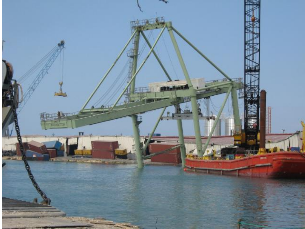
Figure 1.3 Partially submerged container crane at the Port-au-Prince Port (photo courtesy of (Riddle 2010))
