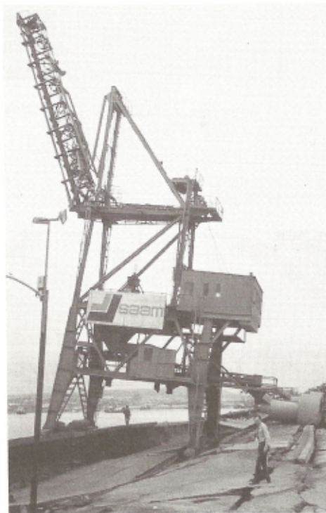
Figure 2.5 – a.) Lateral Spreading: Port de Port-Au-Prince (Photo by (Rix, 2010)) and b.) Crane Settlement: 1985 Chile Earthquake (from (Werner 1998))
