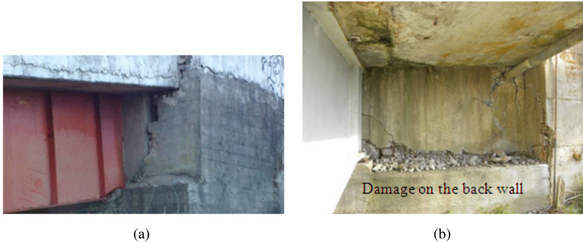
Figure 2.8: Examples of backwall damage (Jibson and Harp, 2011): (a) punching of the Tubul bridge deck into the backwall of the north abutment, and (b) damage at the base of the north abutment backwall of the El Bar bridge.
